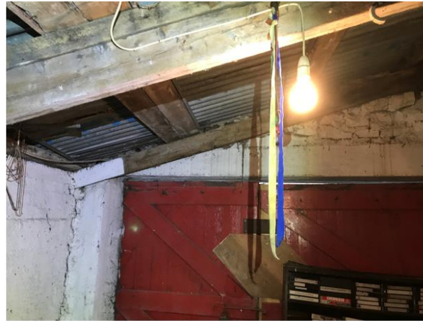
Plate 2: View of internal space of southern shed
