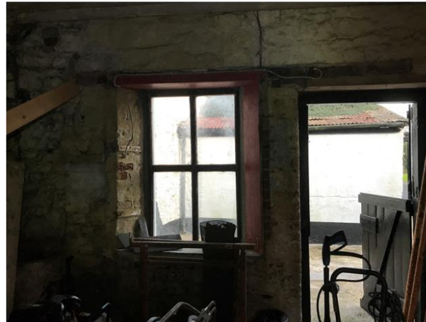
Plate 5: View of window opening of northern shed on north elevation
