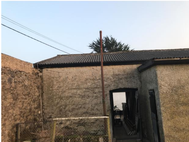
Plate 4: External view of southern shed
