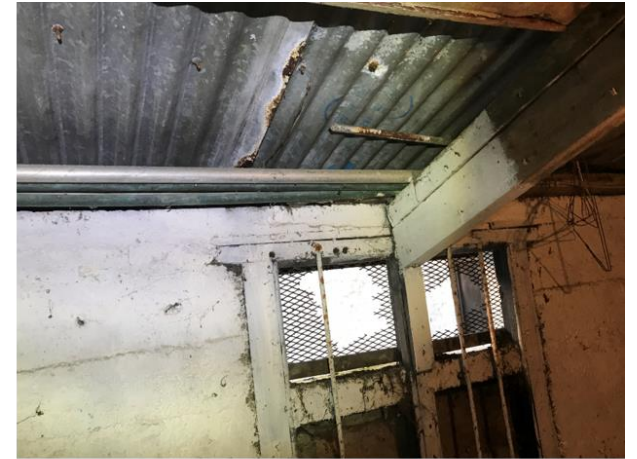
Plate 3: View of window openings in southern shed
