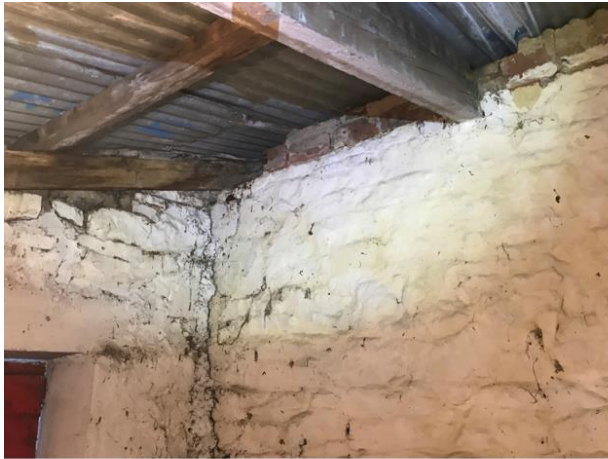
Plate 1: Internal view of southern shed and corrugated roof
