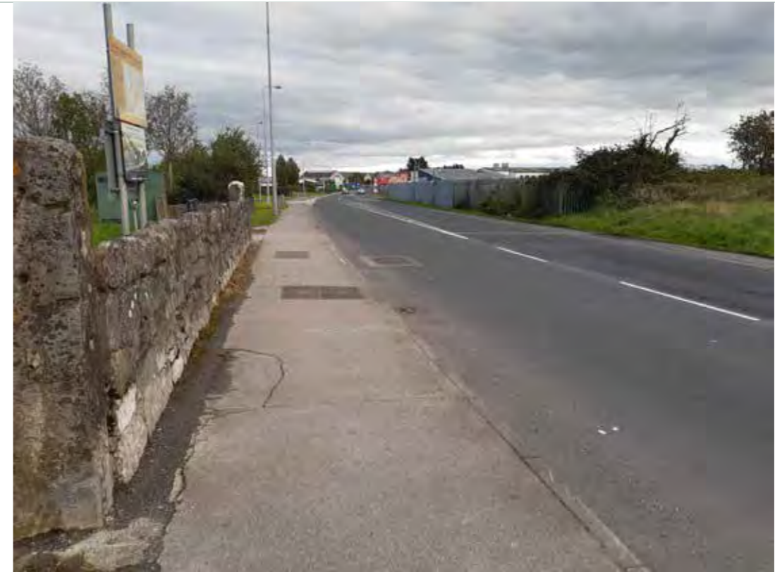
Gap in Footpath on South Side of Station Road
