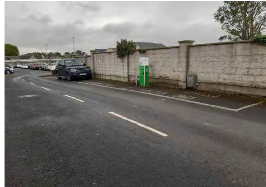
Electric Vehicle Charging Points in Church Street Car Park
