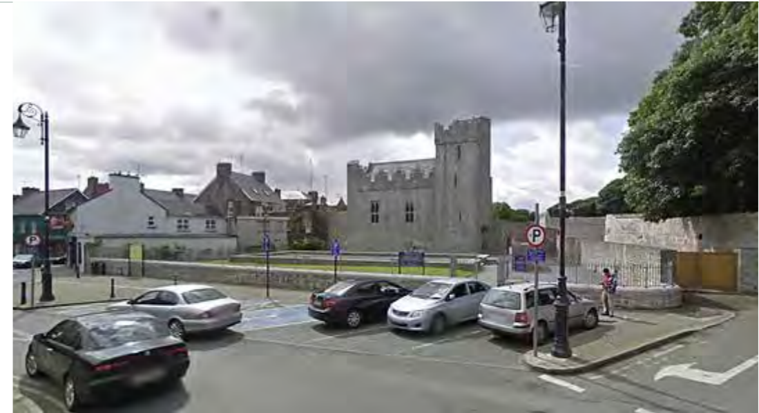
Car Parking and Signage Cluttering Views of Desmond Hall
