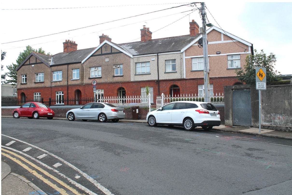
fig 14 Ashbourne Villas at junction with New Street.
