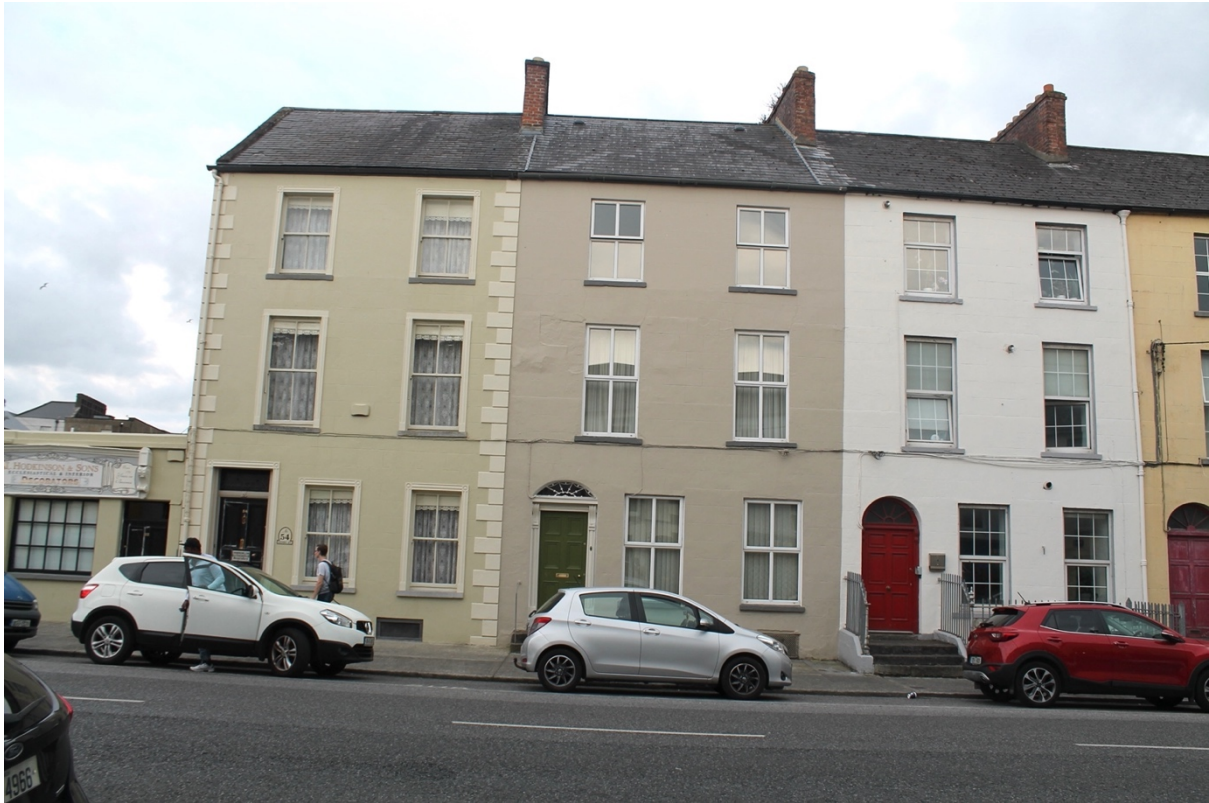
fig 5 54–56 Henry Street, protected structures.
