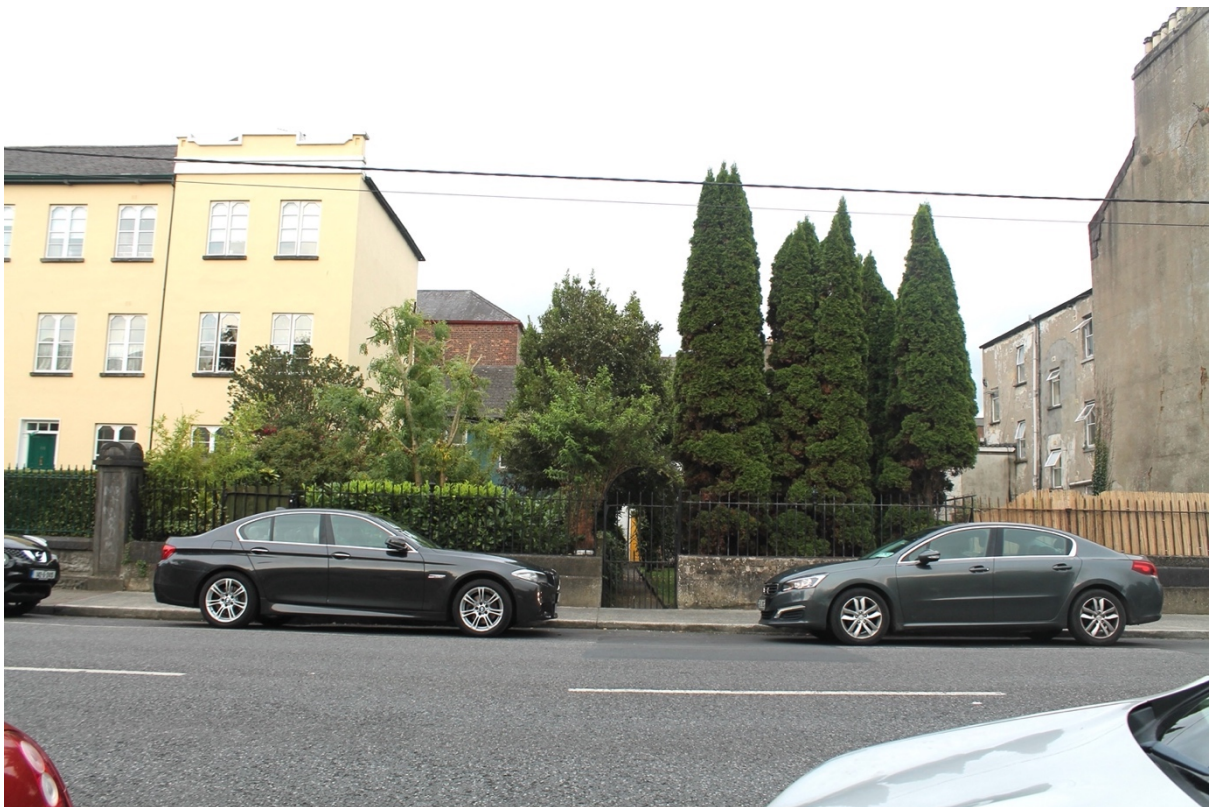
fig 12 Adelaide Terrace, adjacent to Richmond Terrace.
