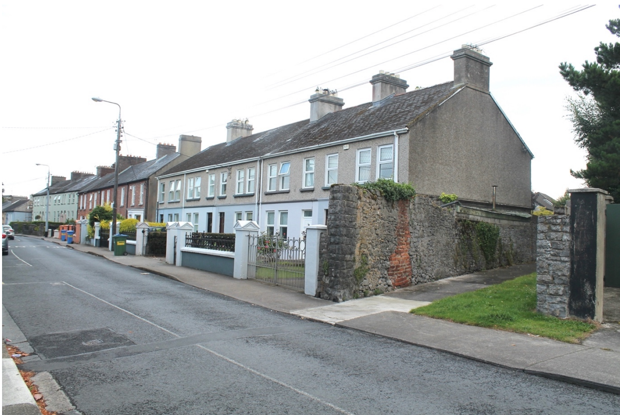
Fig 20 Terraces to east beyond MIC: 20 th -century terrace; Shannoon Terrace; Mount Prospect Terrace.
