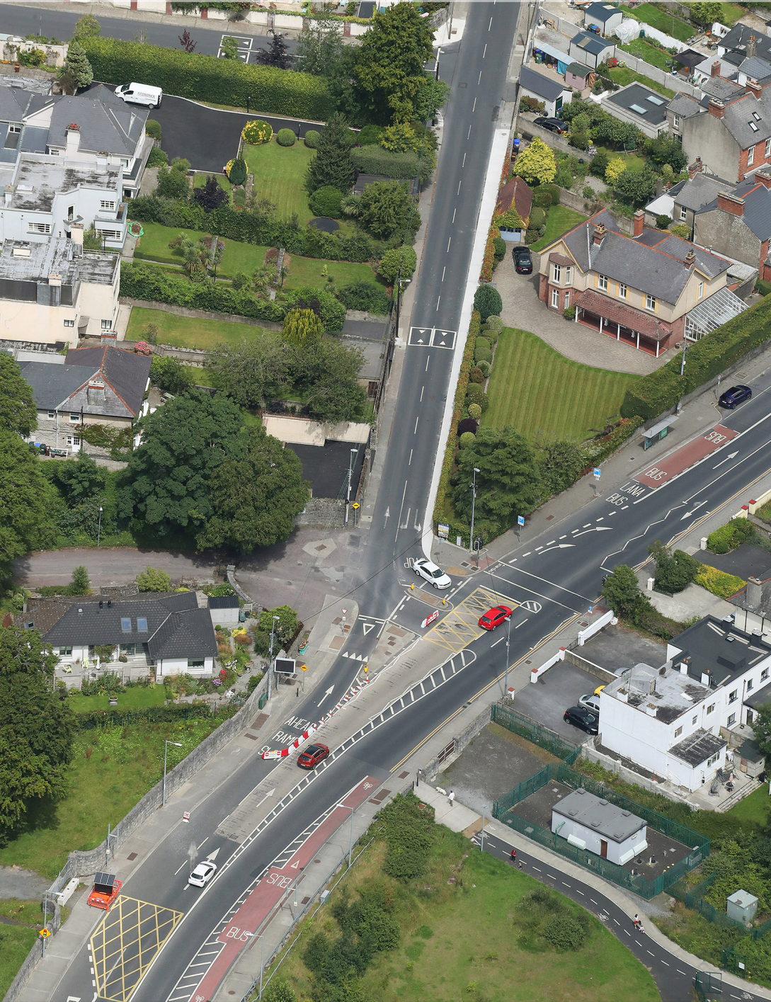
Existing View: Ballinacurra Rd/SCR junction
