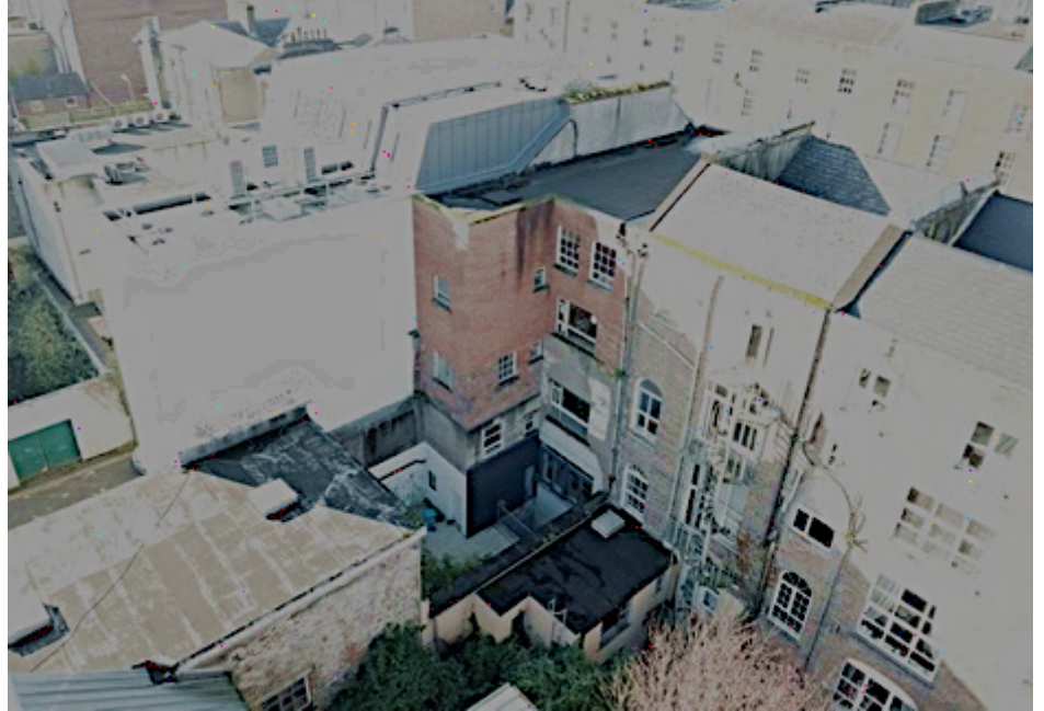
Aerial view of the rear of No. 58 O’Connell Street (red brick building)
