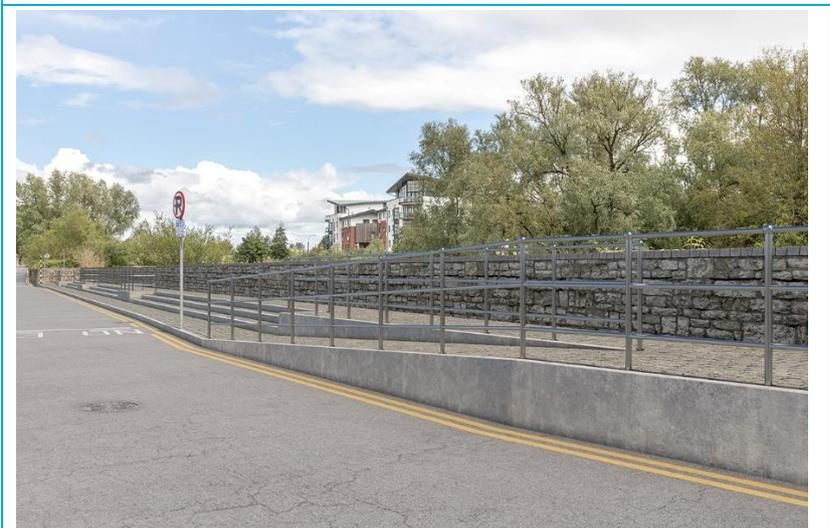
Figure 1-4. Flood defence walls at Sir Harry's Mall
