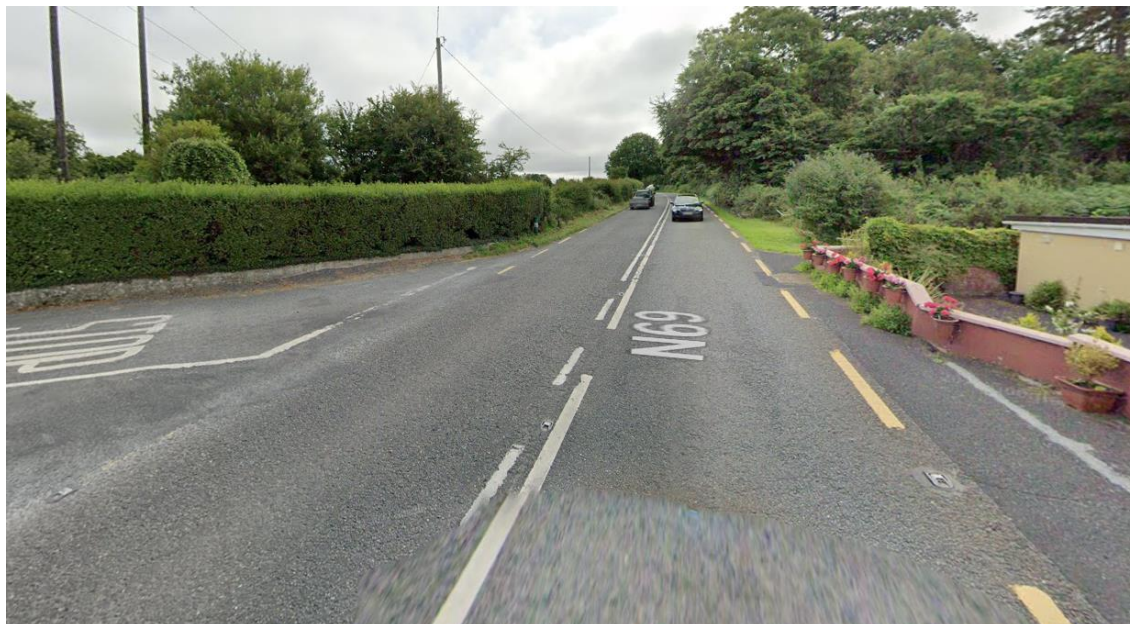
Figure 17: East side view from the junction
