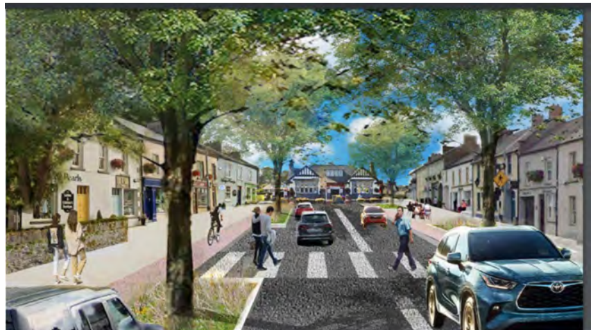
Indicative view of Main St West following public realm upgrade works.
