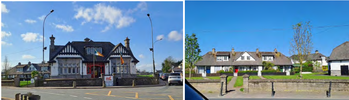
Figure 8.12 Village Hall and adjoining terraced houses
