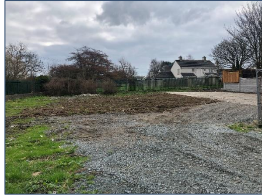
Plate 2-2 View of the concrete foundation (BL3) visible in the top right background. The gravel area (ED1) is visible in the middle and foreground, whilst the exposed earth (ED2) is visible adjacent to the concrete foundation. The recolonising vegetation (ED3) is also visible here in the left background and foreground.
