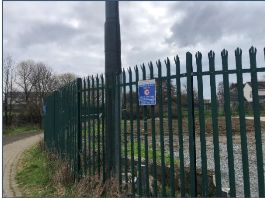
Plate 2-1 View of vacant site with palisade fencing surrounding it and low block wall (BL3) visible in the foreground, and recolonising vegetation (ED3) visible behind this wall and around the base of the palisade fencing.
