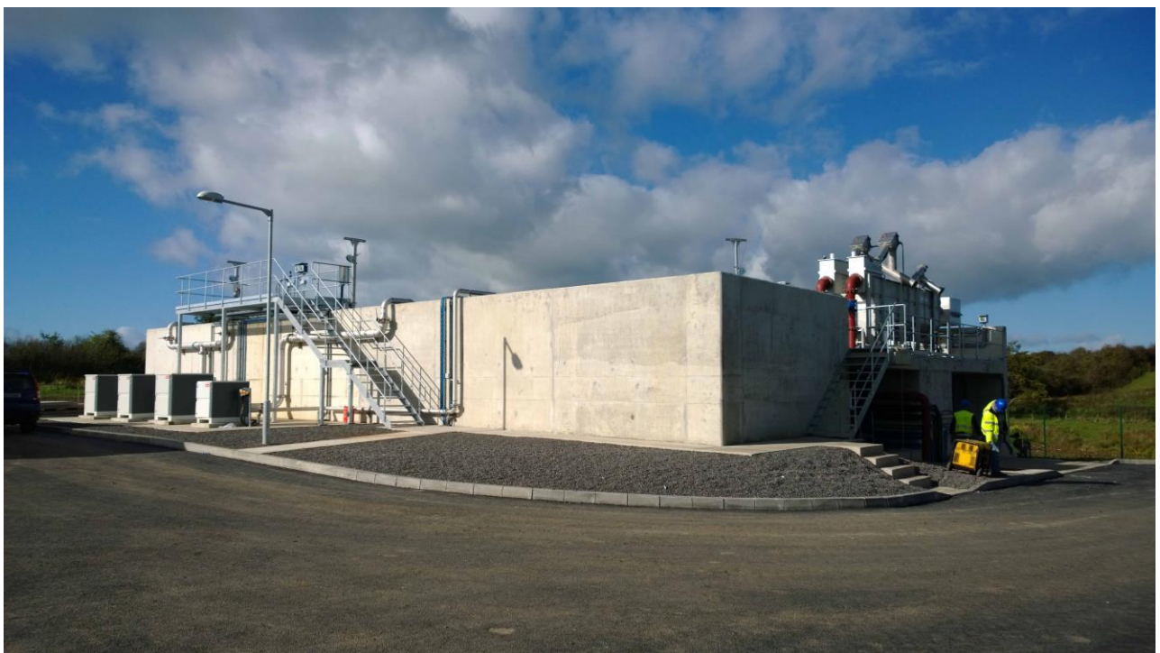
Figure 2: Newly constructed Waste Water Treatment Plant in Kilmallock (Source: Coffey Water Ltd).
