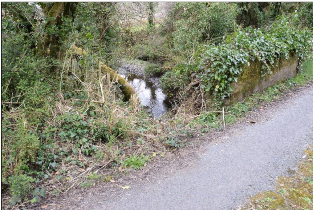
Plate 1 Ballinloughane Bridge over the River Galey in Co. Limerick.
