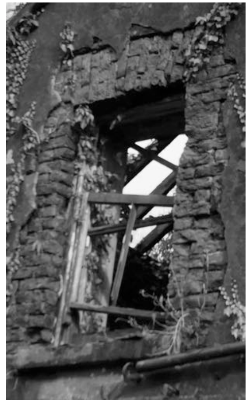
Window reveal detail 2 over 2 sliding sash frames
