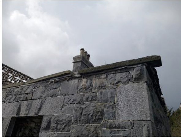
Chimney masonry and wall copings in poor condition
