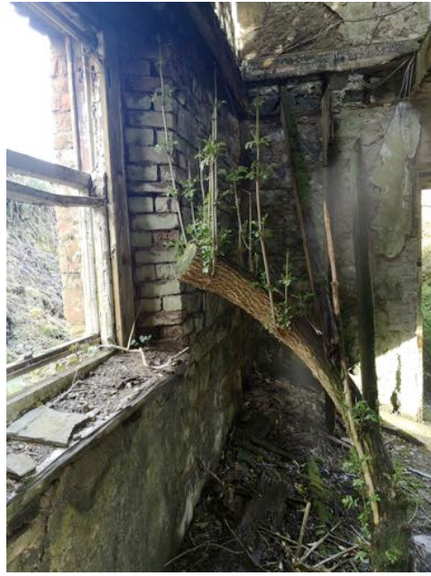
Window reveal detail 2 over 2 sliding sash frames
