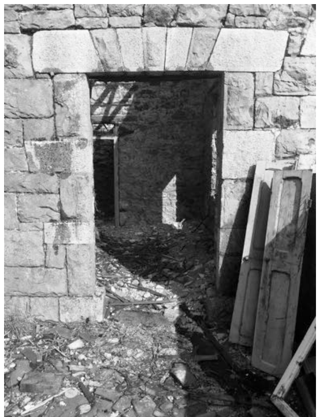
Limestone ashlar masonry in good condition but
