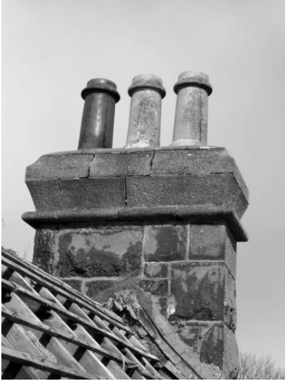
Chimney masonry and wall copings in poor condition
