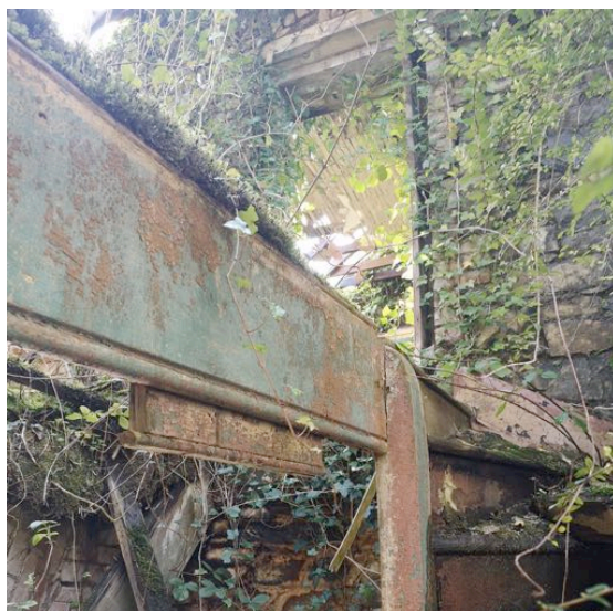
Platform paving Cast iron fire surround Stair / landing detail
