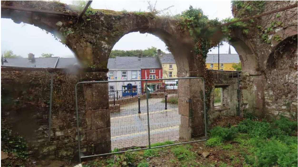
Photograph 002. Internal elevation of front North-West arch wall.
