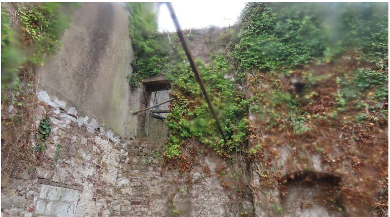
Photograph 005. Internal elevation of South-East back wall.
