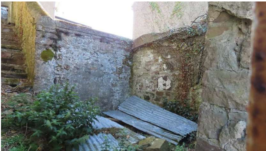
Photograph 025 Yard wall leading to stone steps.
