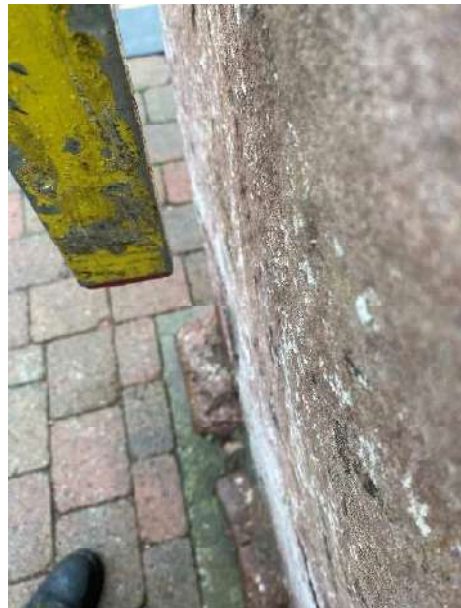
Photograph 024. Gable wall South-West façade the top is leaning outward.
