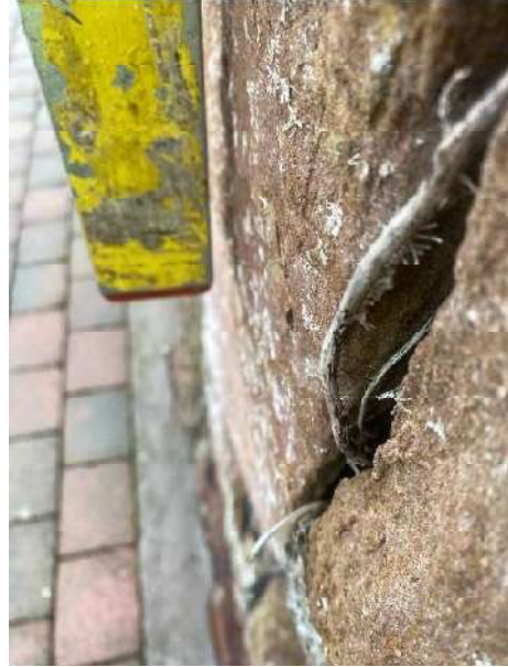
Photograph 023. Front façade facing the square the top is leaning outward slightly.
