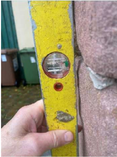
Photograph 025. Gable wall North-East façade the top is leaning outward.
