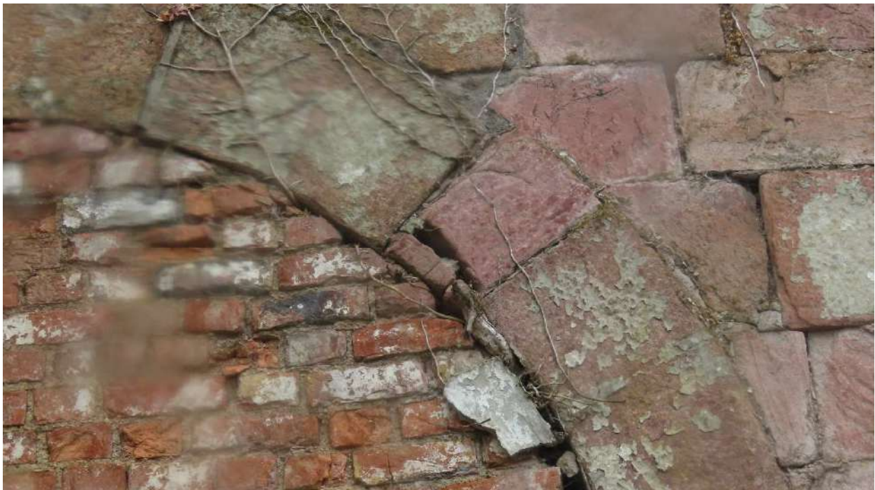
Photograph 019. Showing infilled arch using brick & broken arch stone.
