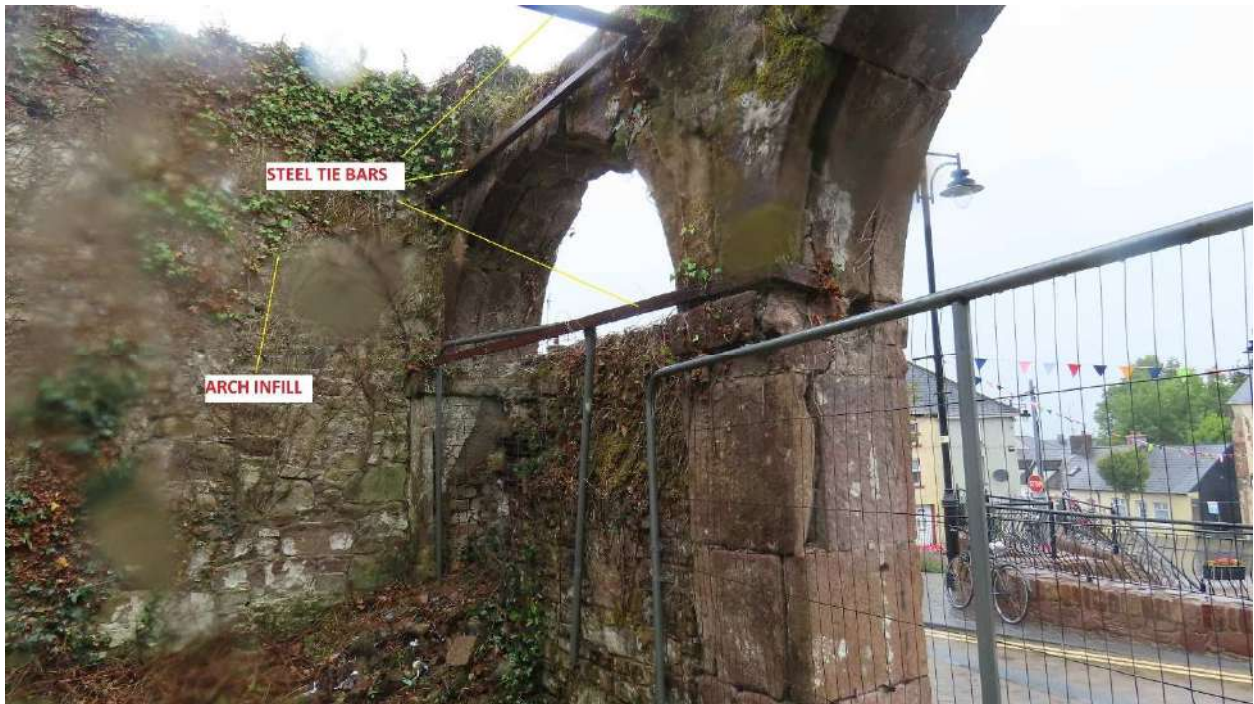
Photograph 014. Steel tie bars
