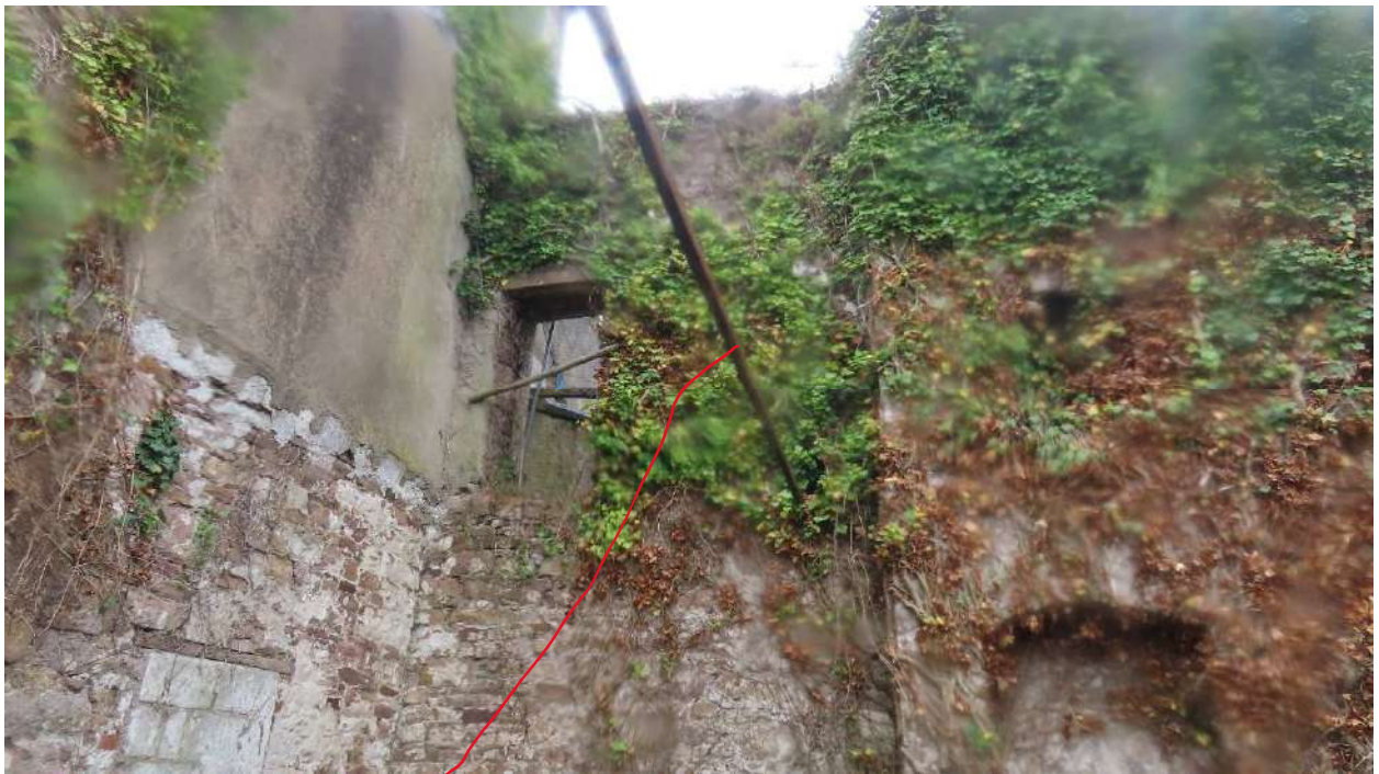
Photograph 013. Steel tie bars.
