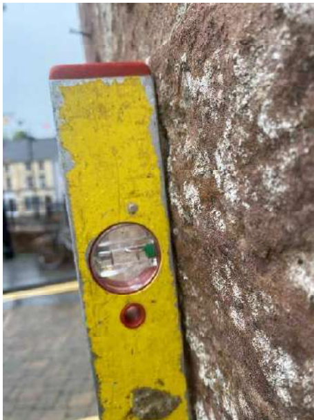
Photograph 024. Gable wall South-West façade the top is leaning outward.
