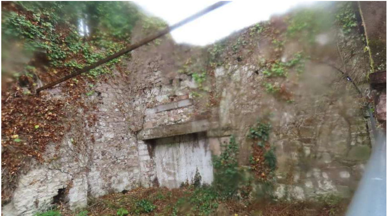
Photograph 004. Internal elevation of South-West wall.
