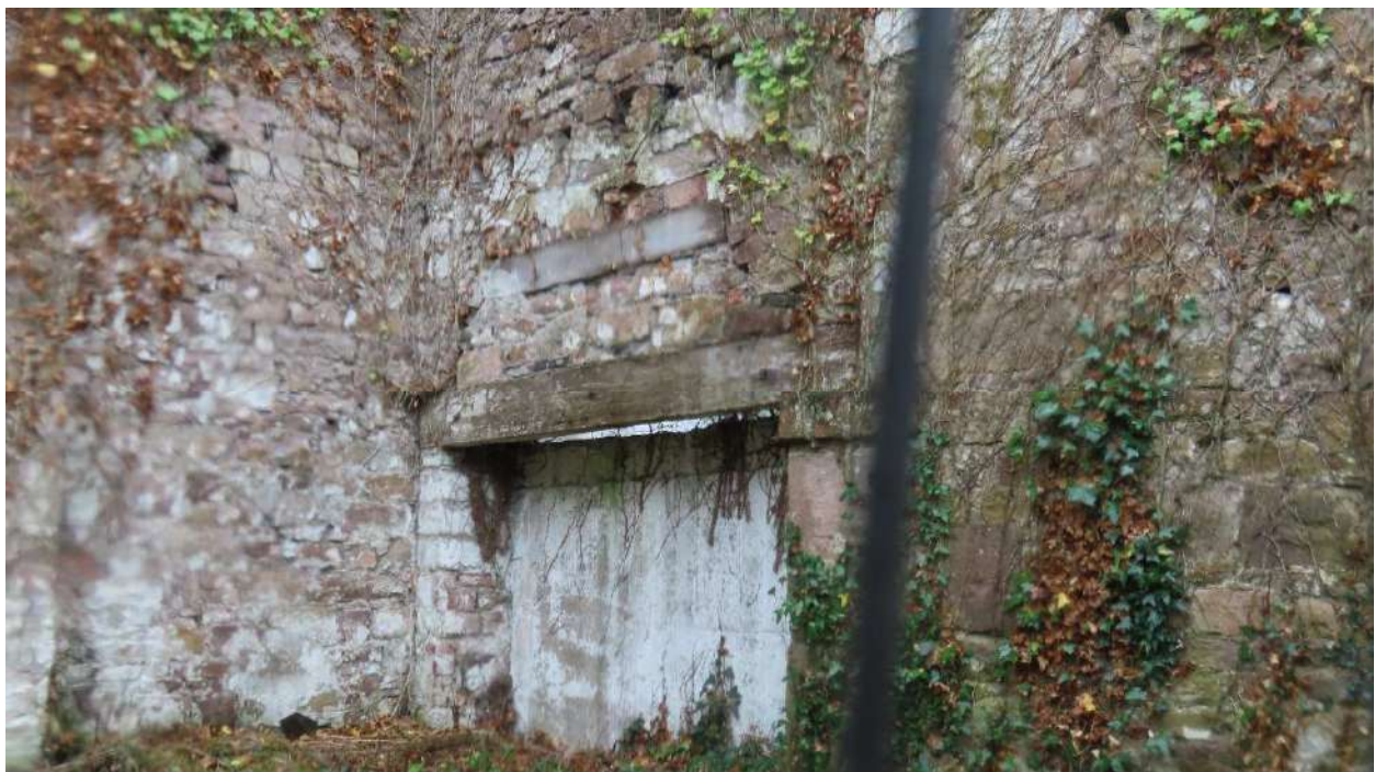
Photograph 015. Timber railway sleeper lintel over opening & concrete infill.
