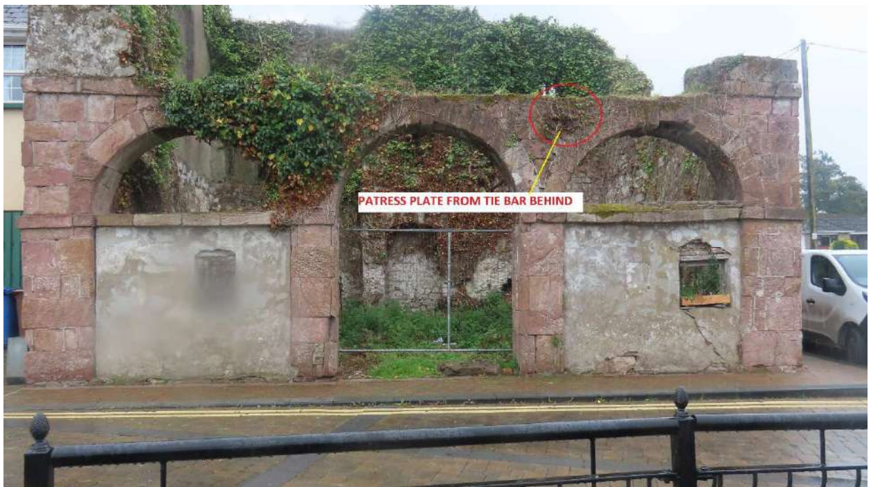
Photograph 021. Showing steel patrix plate from tie bar behind.
