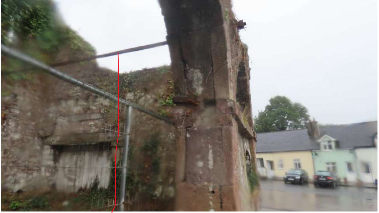
Photograph 012. Steel tie bars.
