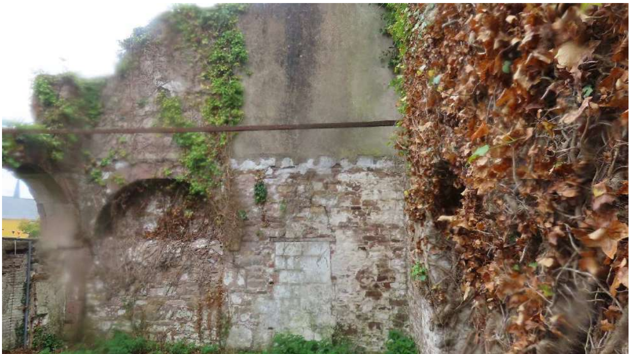
Photograph 003. Internal elevation of North-East gable wall.
