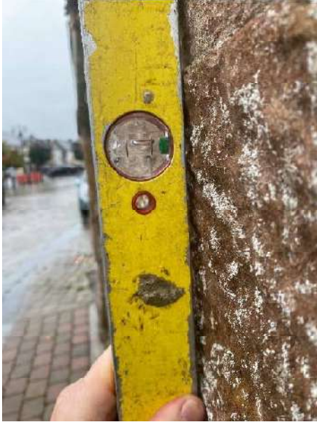
Photograph 023. Front façade facing the square the top is leaning outward slightly.
