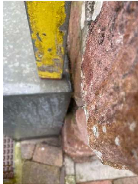
Photograph 025. Gable wall North-East façade the top is leaning outward.
