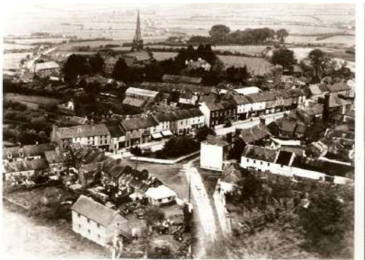
c. 1950 Market House roof appears intact. Former National school on Captains Lane ( now demolished) in foreground.
