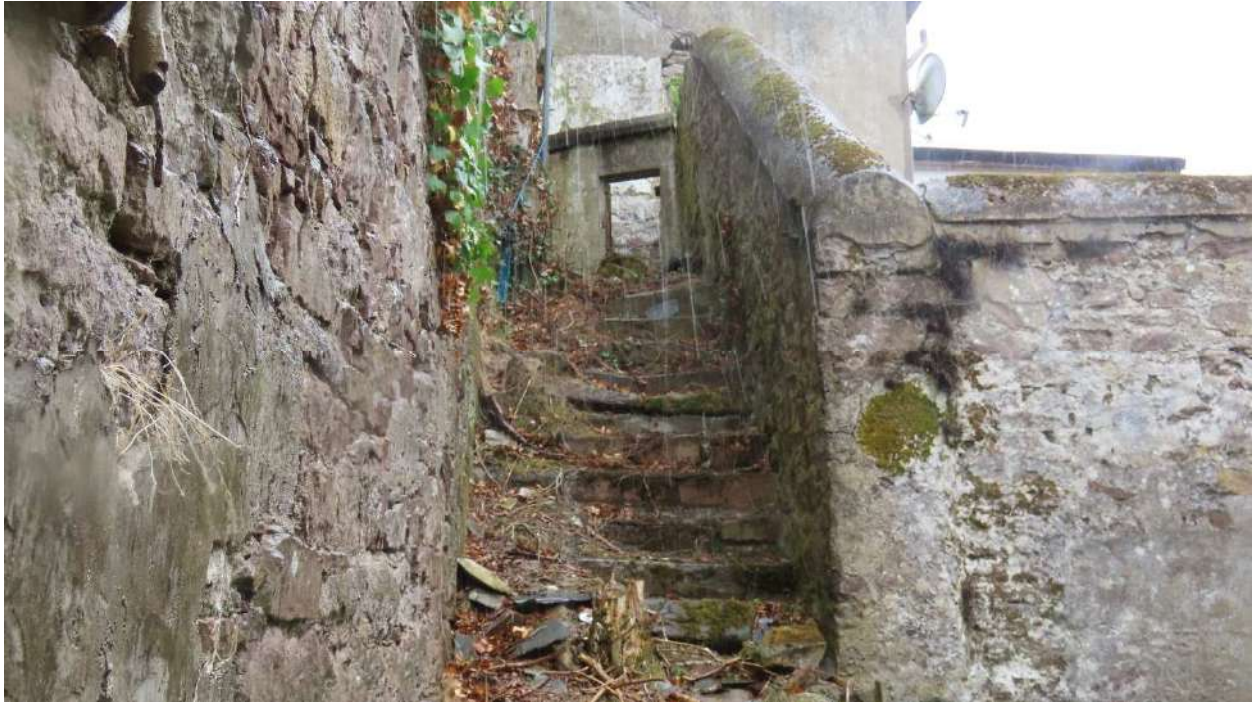
Photograph 008. Back wall & stone steps at the South-East wall.
