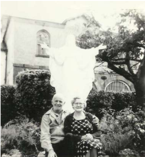
1972 . John Landers with his sister Nora Kenneally at the Sacred Heart Grotto with the Market House in the background. The building appears largely unaltered since 1950 with roof intact. Some deterioration of the rendered eaves detail is evident .
