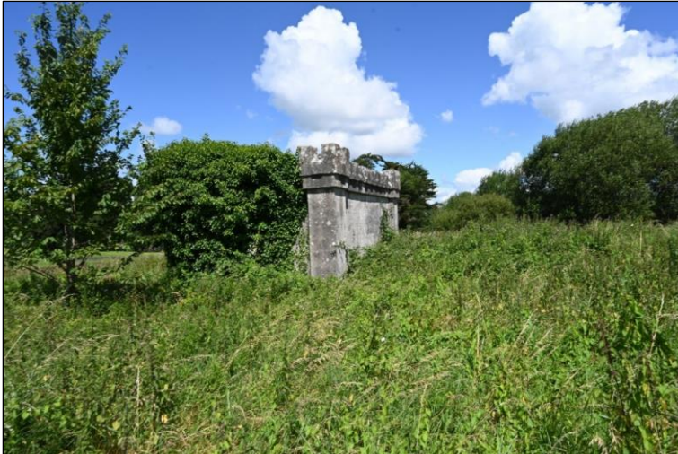
Plate 4 Building located in Field A as indicated in Figure 2. This building has no roof and has low bat potential. No bats were recorded using this structure. Bats forage in this field.
