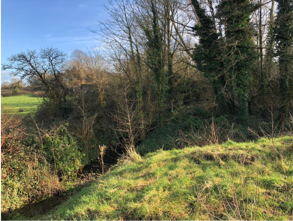
Image 10: Photograph taken from the N69 showing culvert perpendicular to the road flowing north
