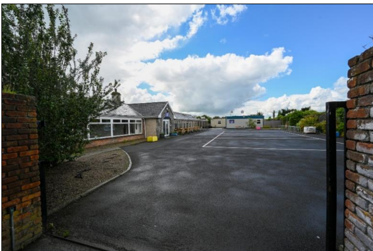
Plate 24 School buildings adjacent to the site – no evidence that they are being used by bats.
