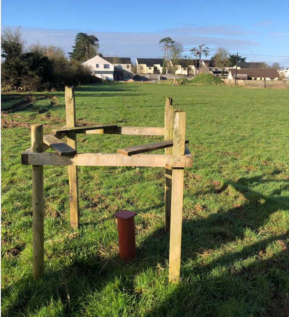
Image 3: Photograph taken of BH205. Wellhead is secure with protective fencing erected.
