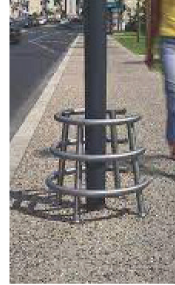
Lighting column protection for lamp posts in shared surface spaces
