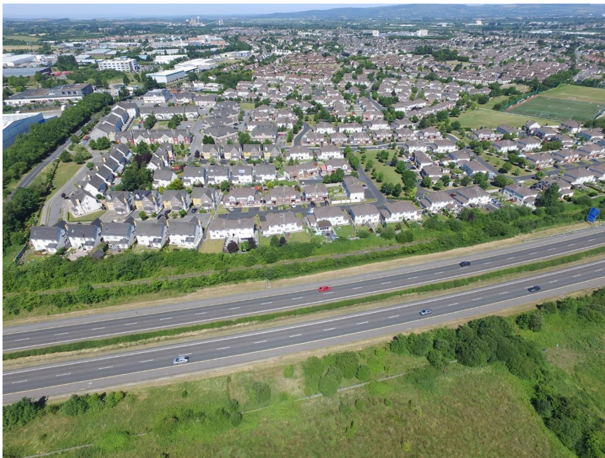
Figure 3.4. The M20 motorway adjacent to Ballycummin (Hotspot 11).
