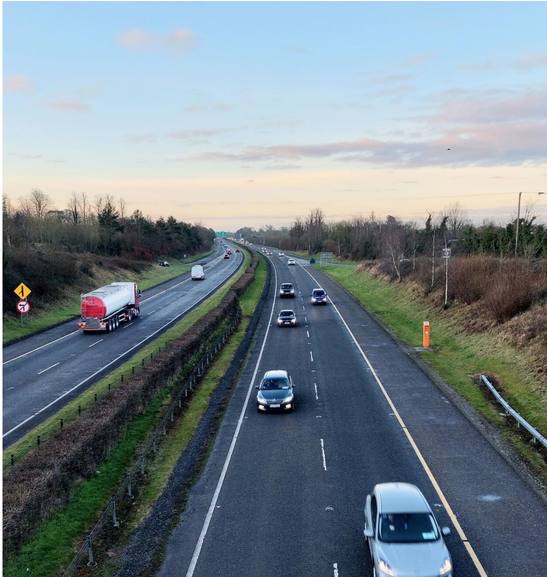
Figure 3.1. Section of M20 motorway south of Junction 4 adjacent to Patrickswell.
