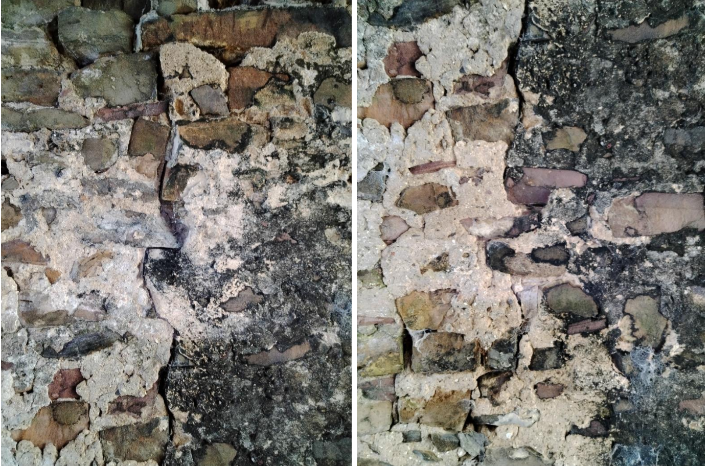
Figure 2. Longitudinal cracks in the arch barrels.
