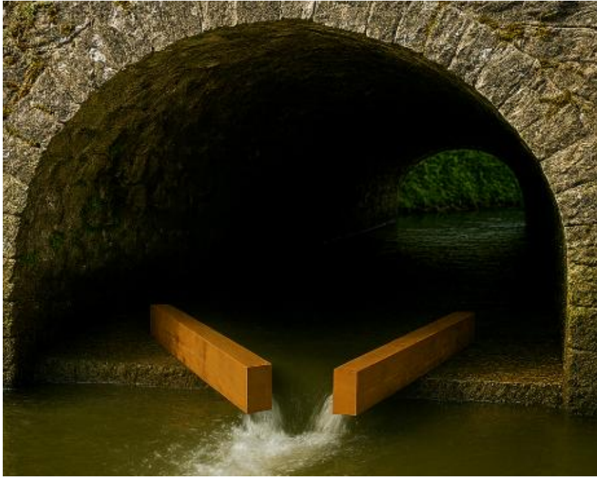
Image 4-1 – Proposed layout to baffles under arches
