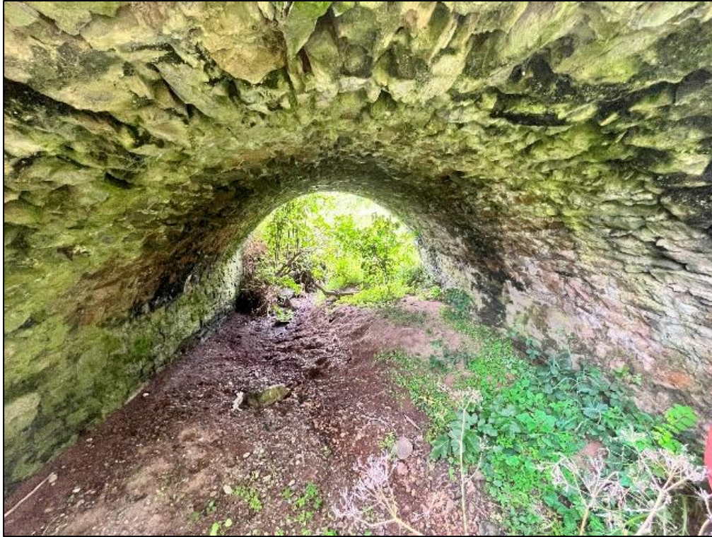
Image 2-1 – Arch 4, south arch of bridge
