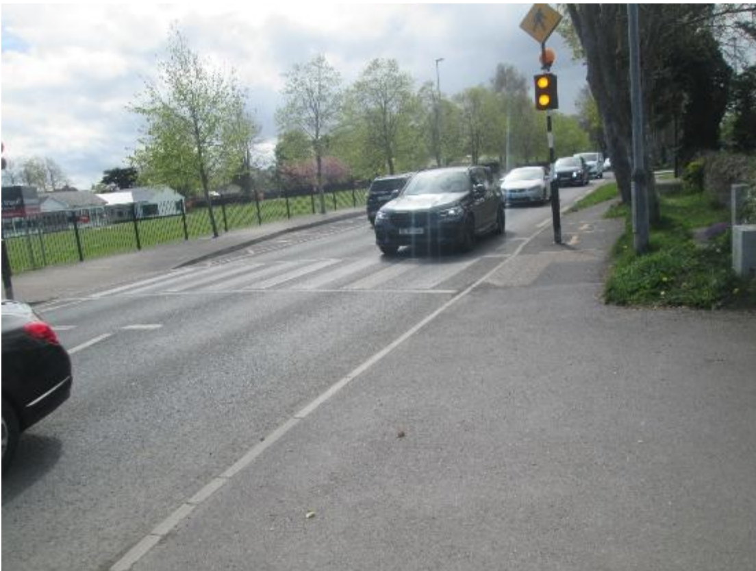
Figure 5.8 Photo 8 Existing Pedestrian Crossing at Scoil Naomh Iósaf
