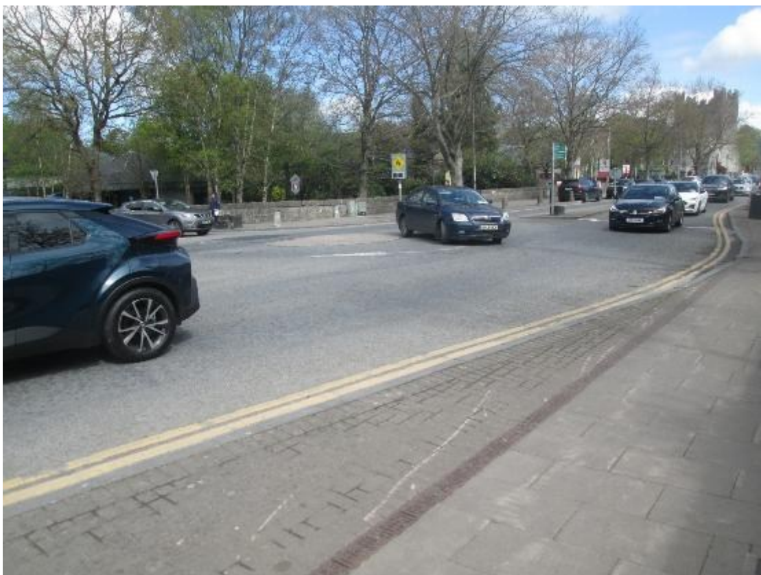
Figure 5.10 Photo 10 Existing Roundabout at Main Street / Station Road Junction
