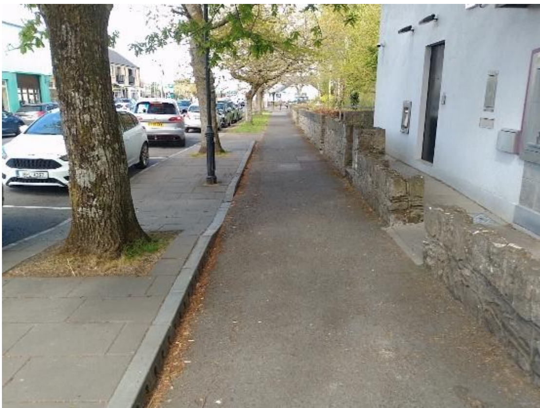
Figure 5.14 Photo 14 Existing Linear Drainage Kerb and Footpath
