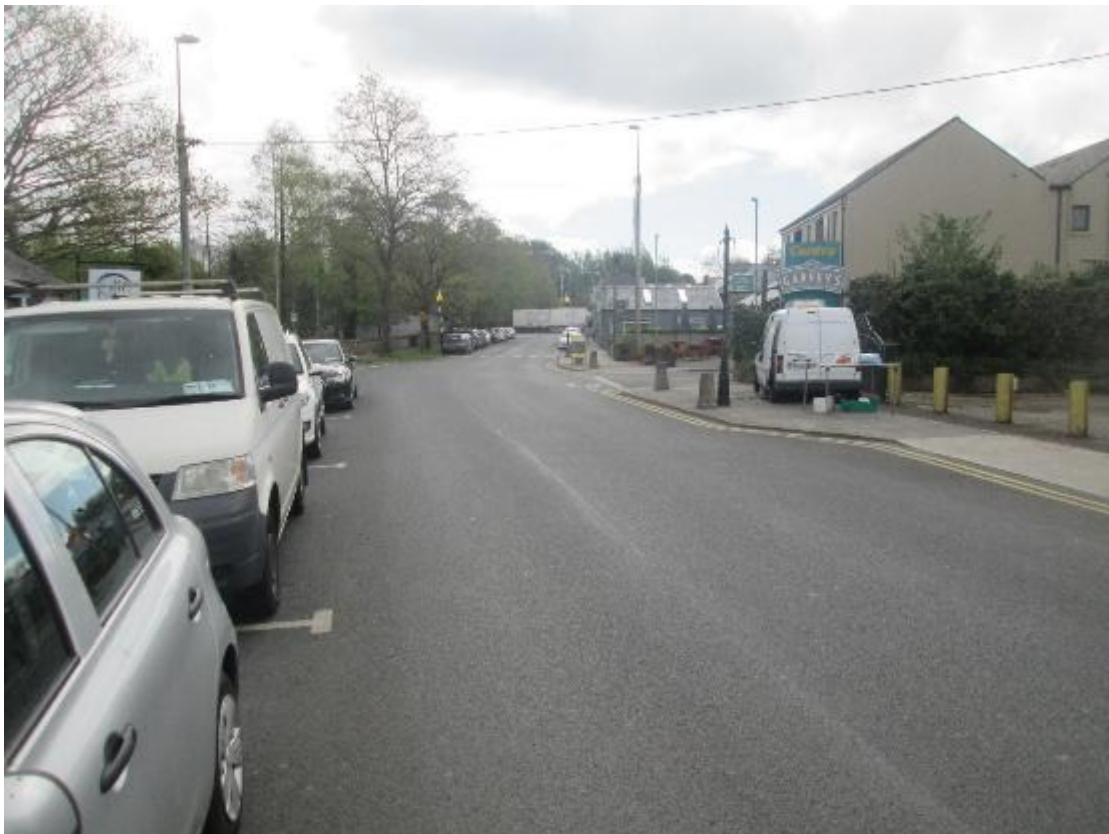
Figure 5.2 Photo 2 Station Road (South)
