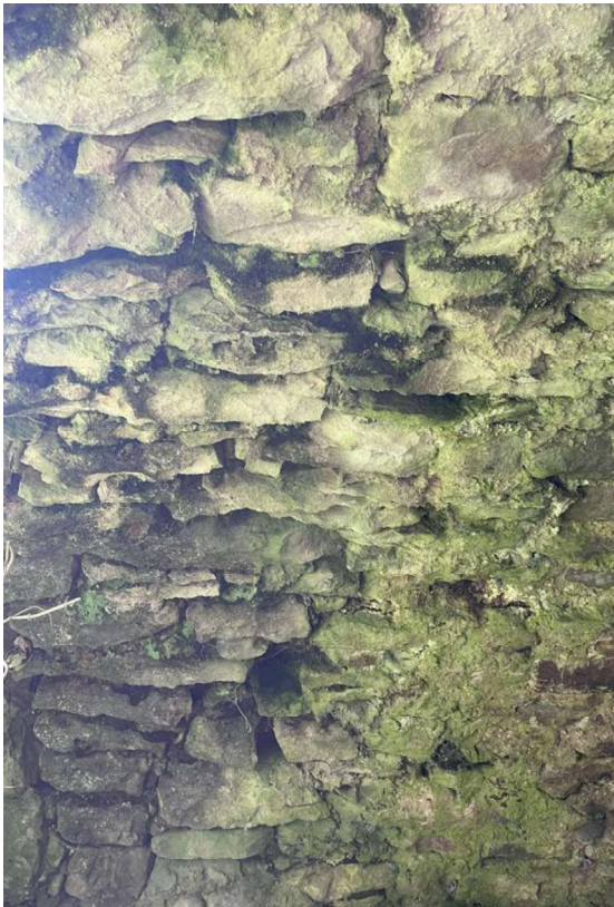
Image 3-4. Cracks, holes and dislodged mortar on the underside of one of the arches.
