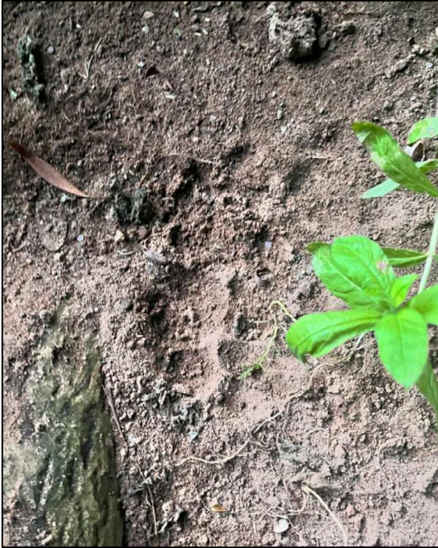
Image 2-4 – Survey 2 – Dog prints under arch 4 of bridge
