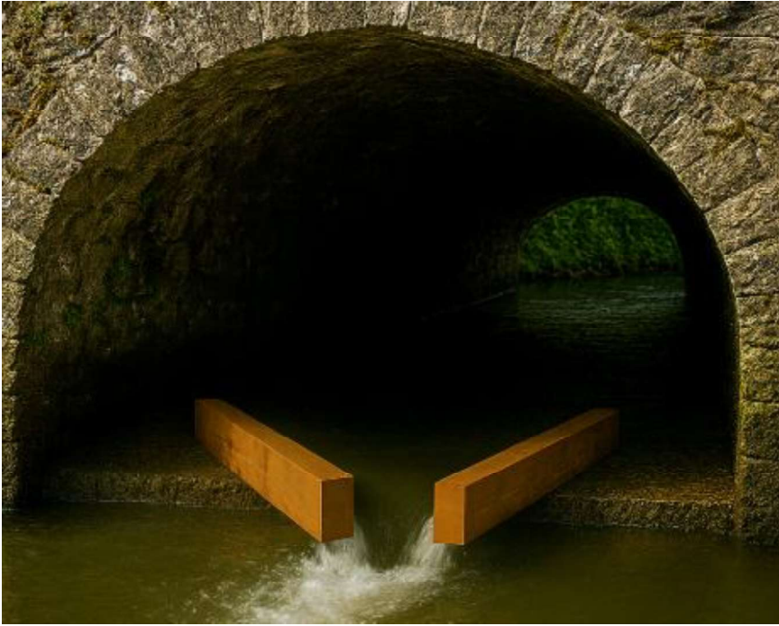
Image 7-1 – Proposed layout to baffles under arches
