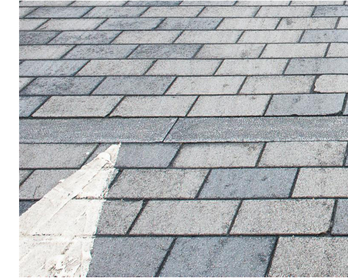
PCC paving slabs (to match Link Street crossings) at crossing locations around Main Square
