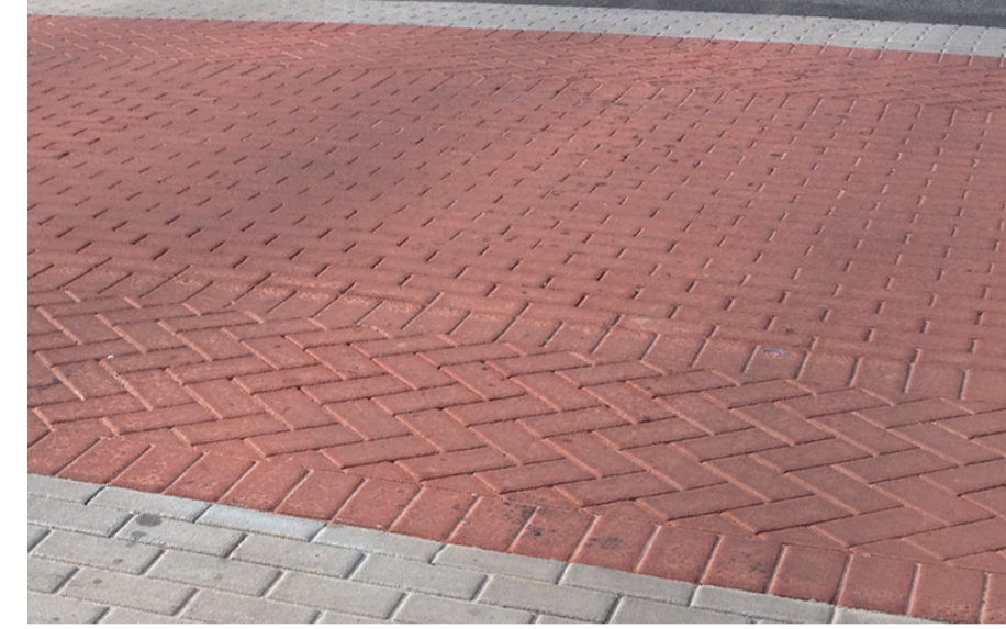
Imprinted asphalt to raised tables
