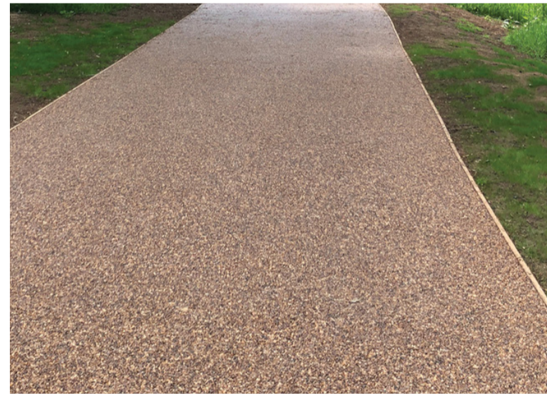
Resin bound paving to formalised greenspace paths
