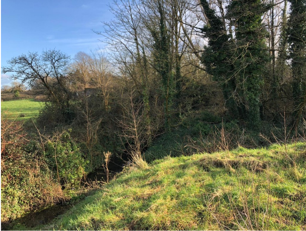
Image 10: Photograph taken from the N69 showing culvert perpendicular to the road flowing north
