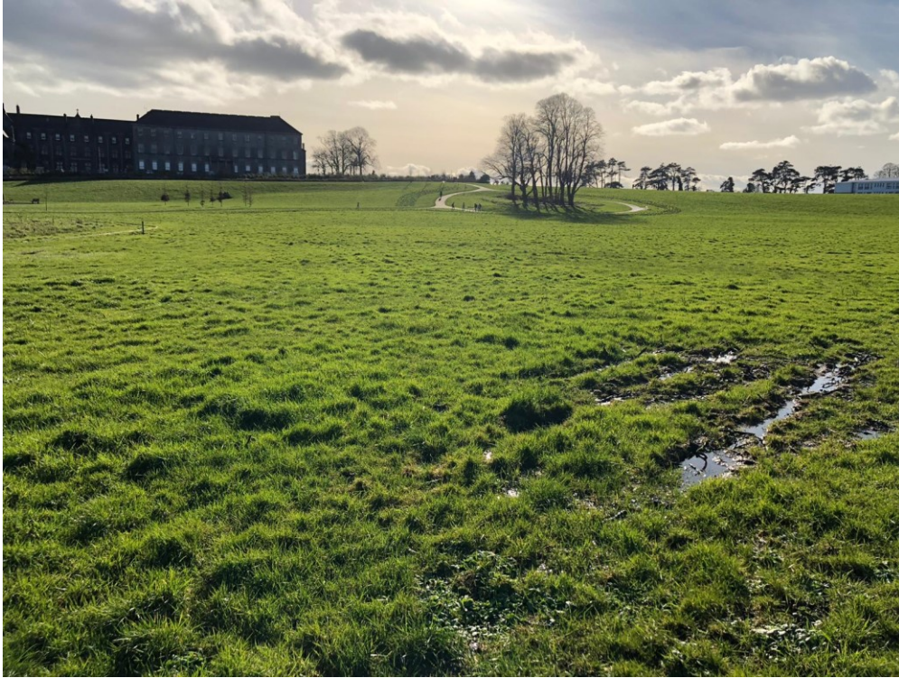
Image 8: Photograph taken in Mungret Park. Ponding observed in the lower gradients of the site.
