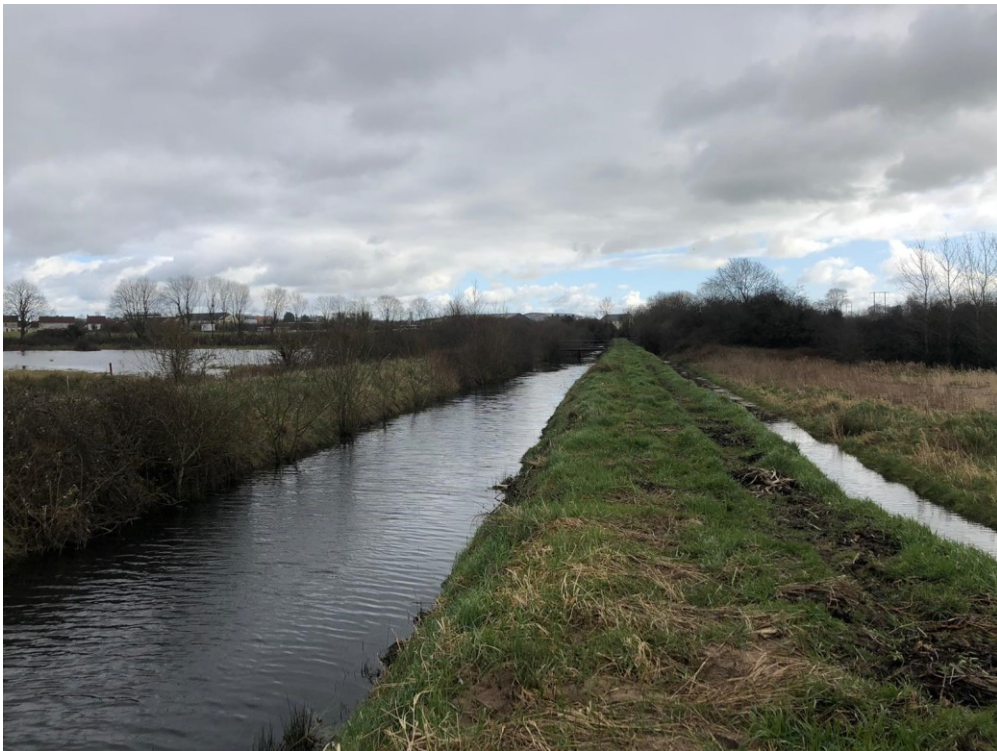
Image 5: Water features from left to right: turlough, manmade canal and toe drain.
