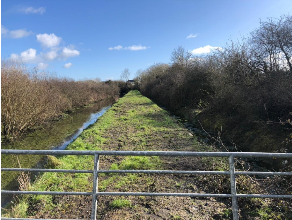
Image 4: Photograph of manmade canal and toe drain
