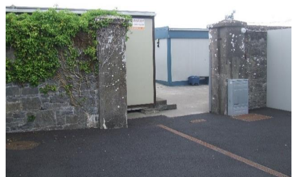
Fig.10 Survey photo Wall (C) Piers to be retained
