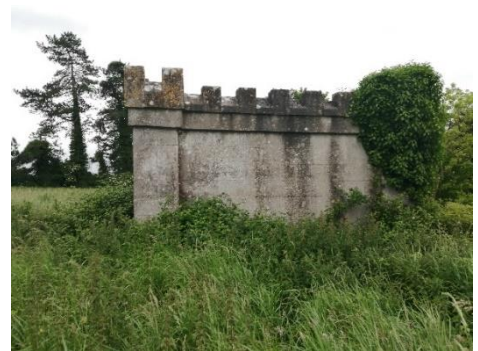
Fig.11c Survey photo: Observatory North Facing Elevation
