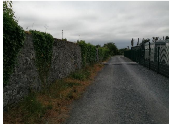
Fig.07 Survey photo of Outer wall (B) West Boundary
