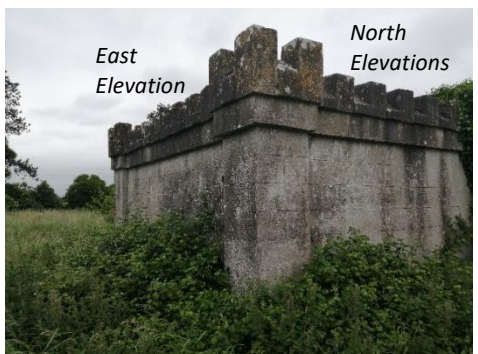
Fig.11f Survey photo: Observatory East & North facing Elevations
