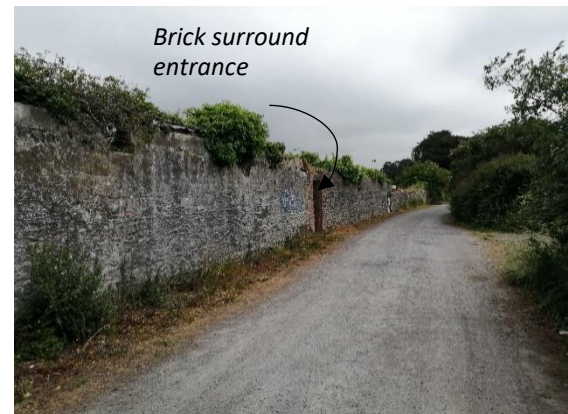
Fig.08 Survey photo of Outer wall (A) South Boundary
