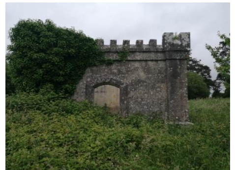
Fig.11e Survey photo: Observatory West facing Elevation
