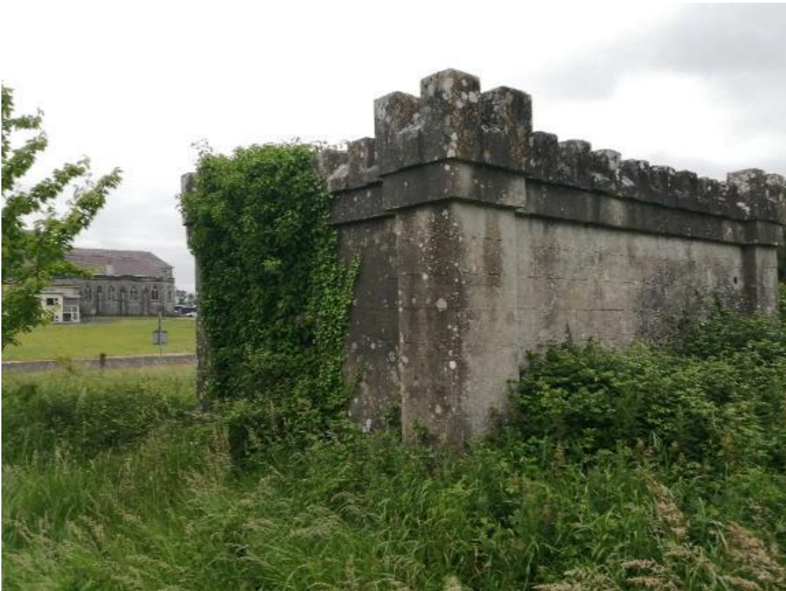
Image 4: The existing visual relationship between the College and the Observatory would be retained. (Read in-conjunction with Conservation Report; RP-A-1510)
