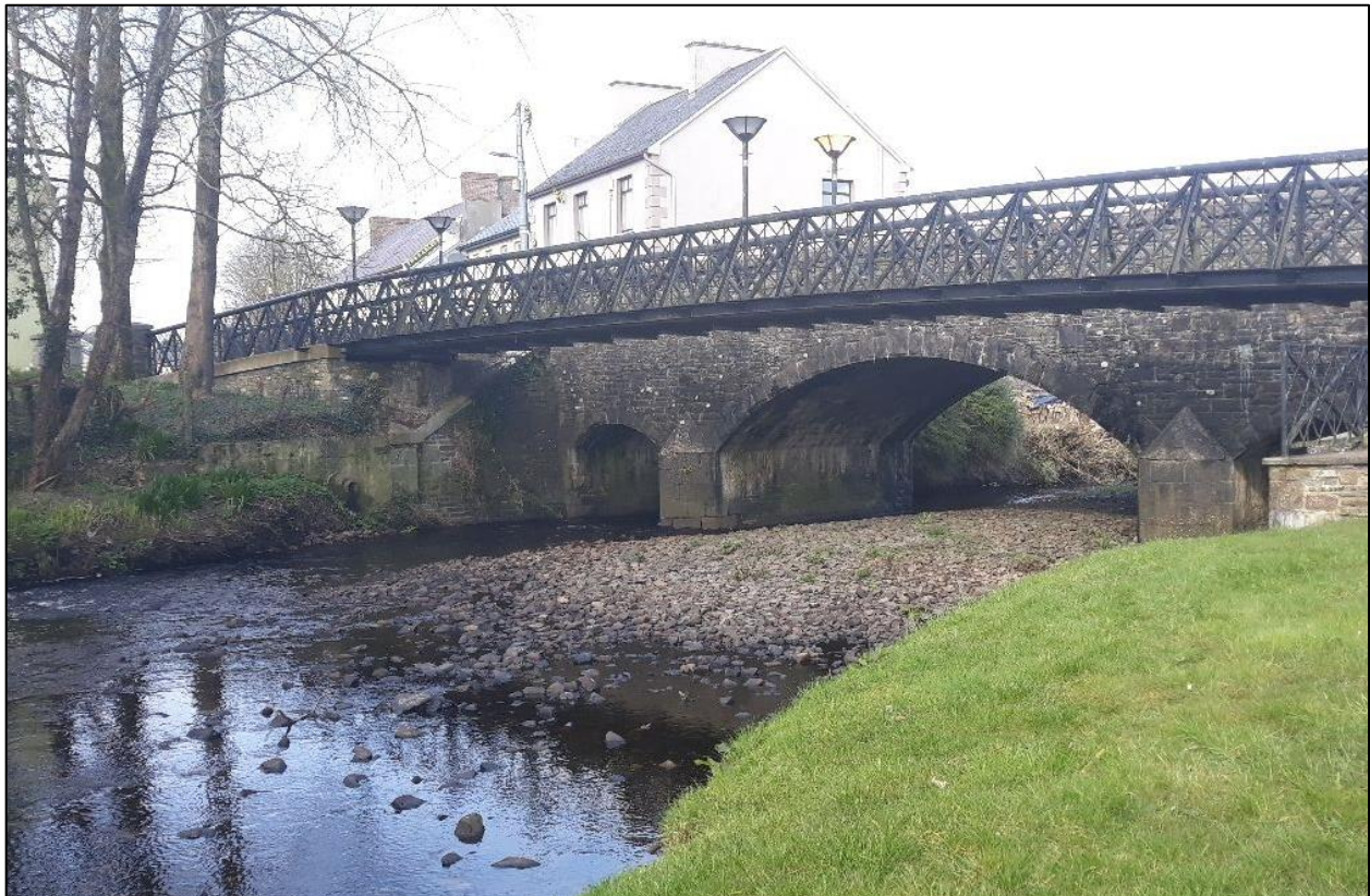
Figure 1-1: Gravel deposit upstream of Athea Bridge (Taken on 05/03/21)
