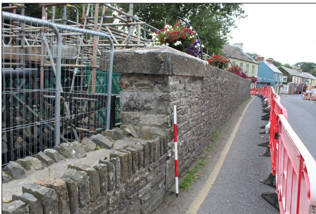
Plate 7: Parapet wall of Athea Bridge, taken from east.
