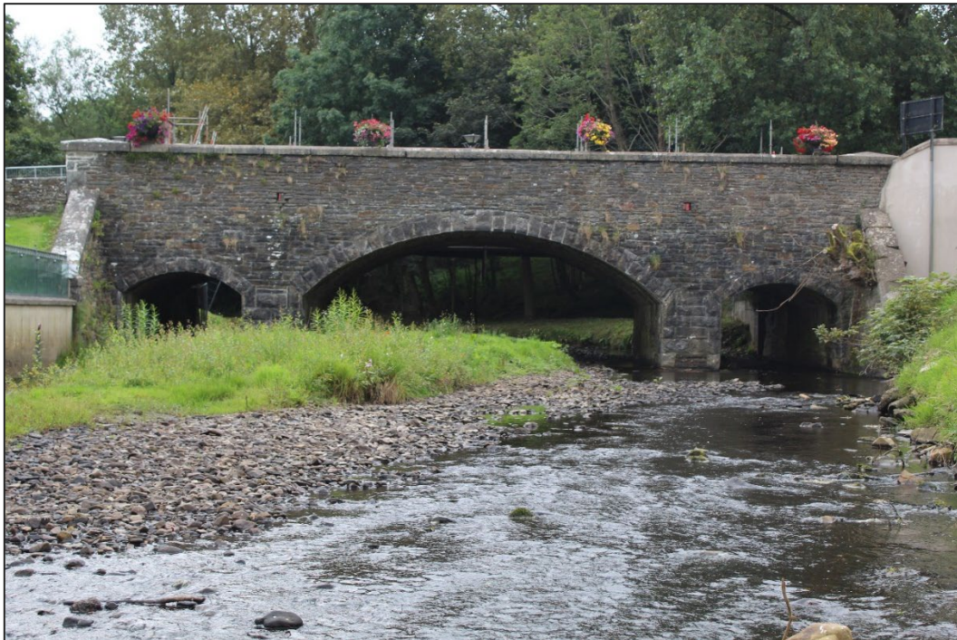
Plate 6: View of Athea Bridge northern elevation, taken from the north.
