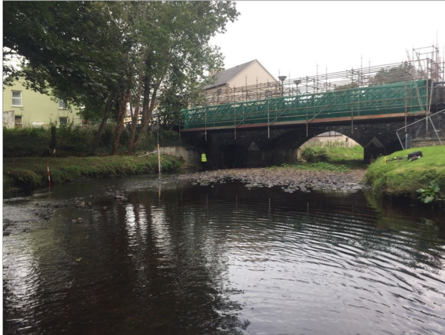
Plate 1: Visual survey and bridge recording in progress, taken from southeast.
