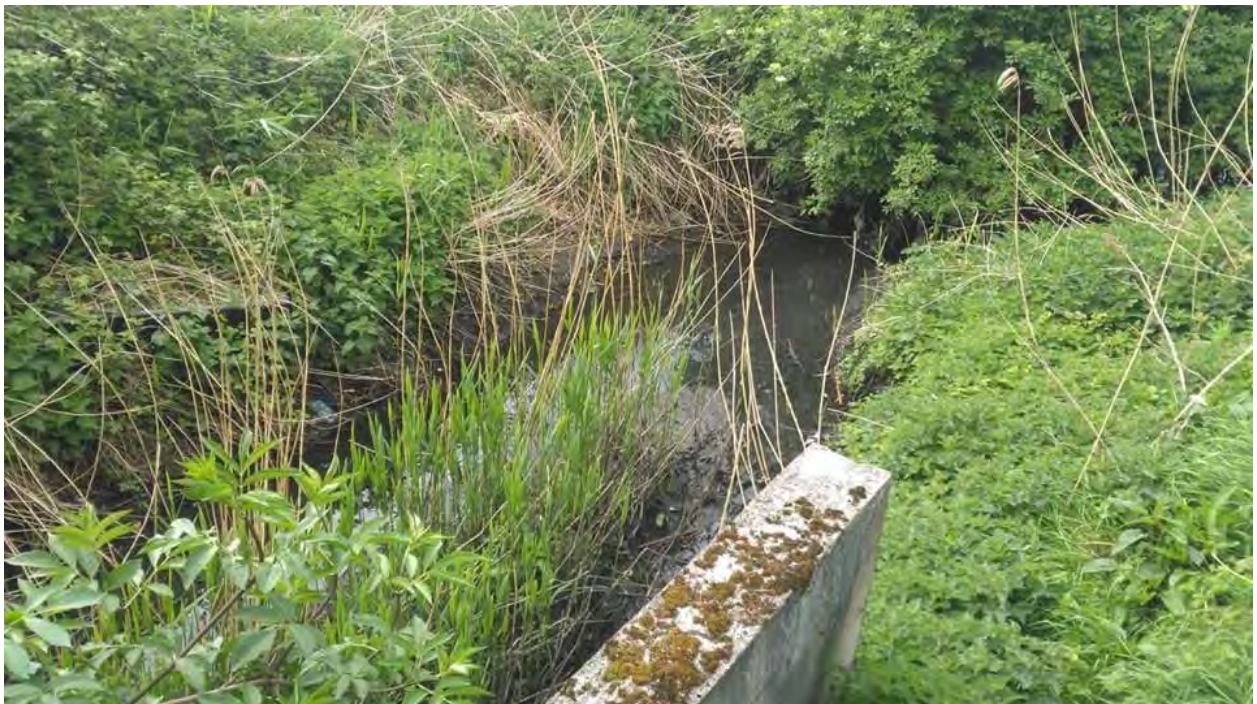
Image 2: Picture of OPW Arterial Drainage Channel and headwall
