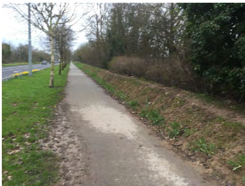
Plate 2 More recently raised embankment (in 2015) along the Condell Road in front of Ted Russell Park
