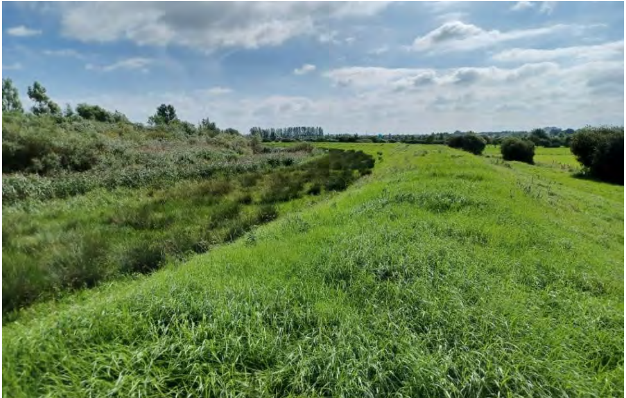
Image 3: Existing flood defence bordering Ballincurra Creek to the east of site 3
