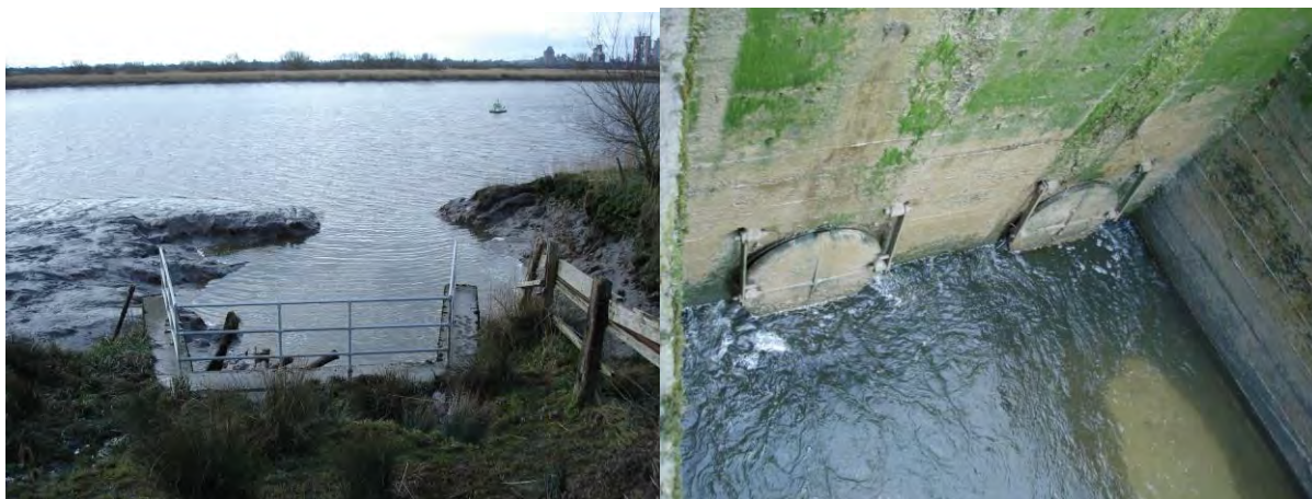
Plate 1 Flapped outfall to Shannon Estuary - twin 600mm diameter pipes
