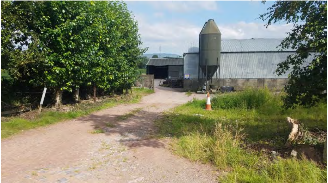
Image 5: Existing farmyard in site 2 (east)
