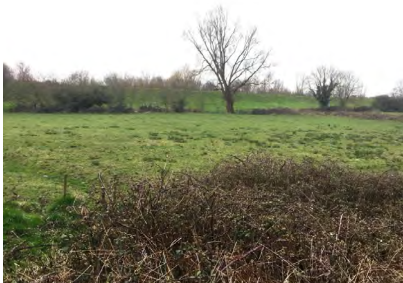
Plate 3 Section of OPW Flood Embankment in background protecting the Clonmacken Area
