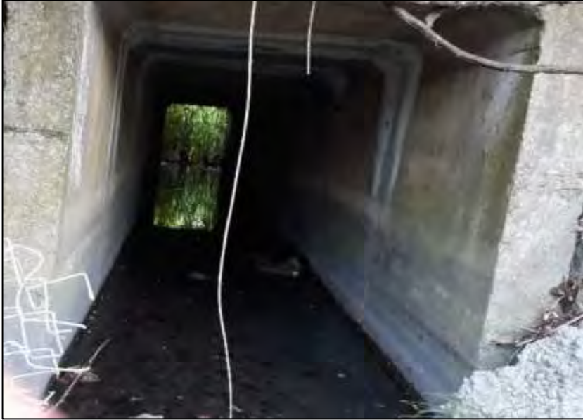
Photo 3: Location A – Crescent Shopping Centre drainage outlet
