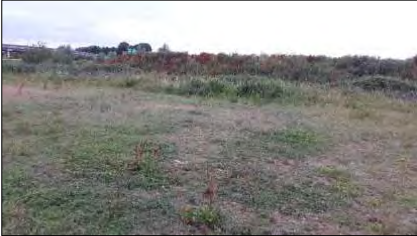
Photo 12: Location B – Drainage culvert exit
