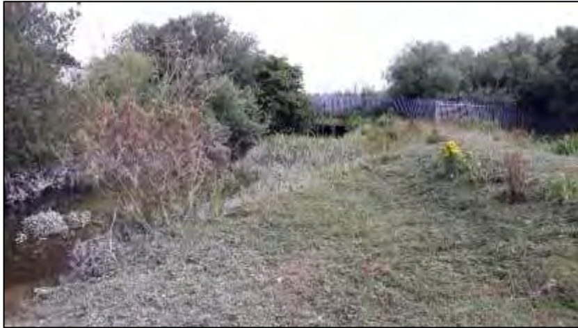
Photo 18: Location F – Railway crossing (Structure 3965) facing upstream
