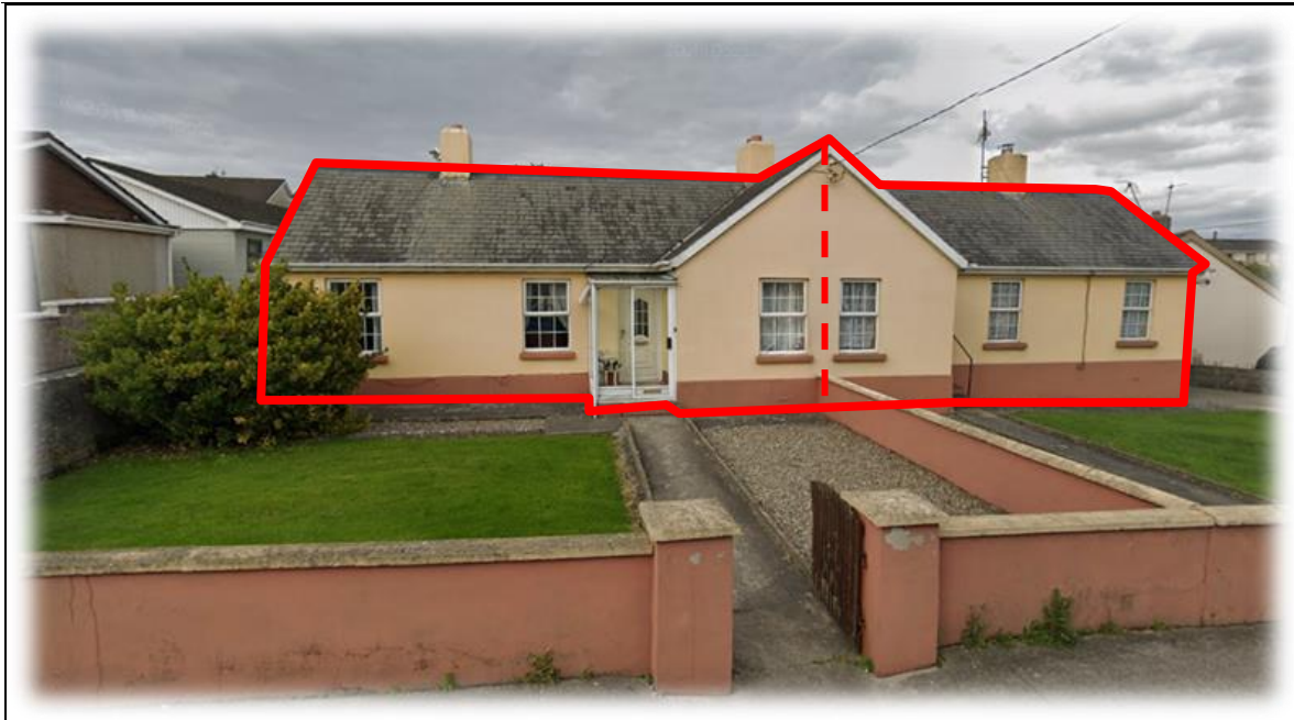
Figure 2 Photo of site - red line denotes the two houses and the dashed line the approx. division of No.1 and No.2 St. Mary's Terrace.
