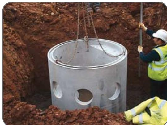
Figure 19 - Checking Orientation/Level of Chamber
