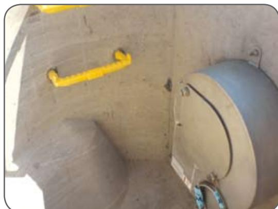
Figure 21 - Close up of Hydro-Brake® Flow Control within Chamber
