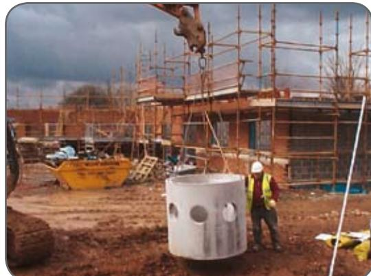
Figure 16 - Chamber being lowered into position.
