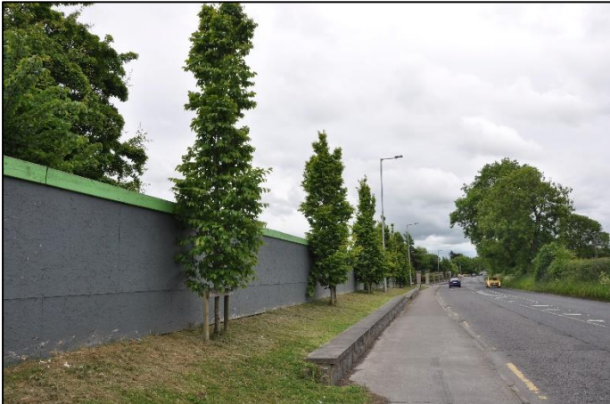
Plate 4 Recently planted ornamental vegetation and retaining wall which will be removed as part of the proposed development. This vegetation will be replanted.
