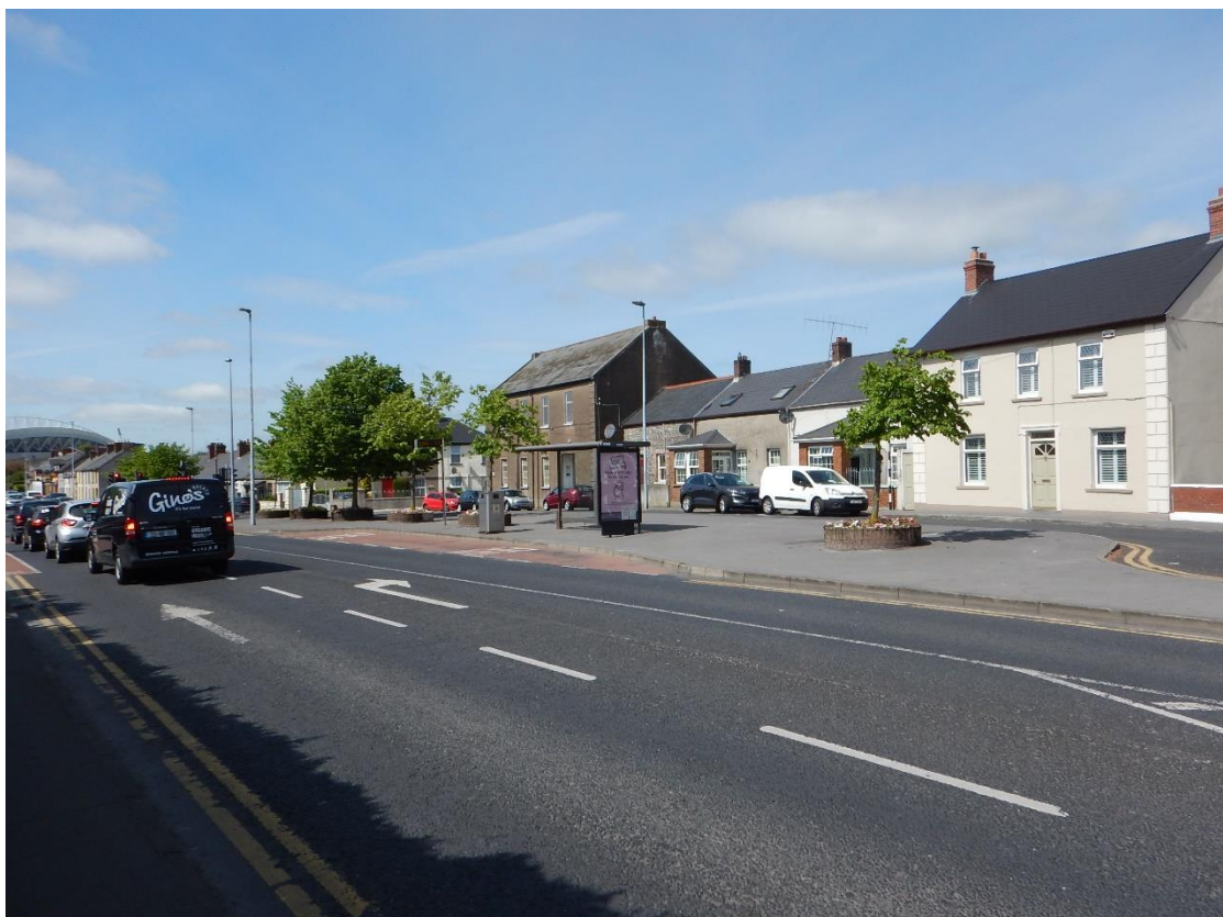
6. Young Lime trees (T56-63) planted into a series of raised beds/planters along High Road
