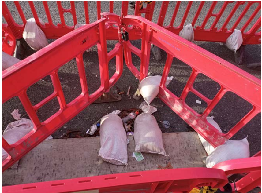
March 2022 – Stone slabs falling through road hole into cellar
