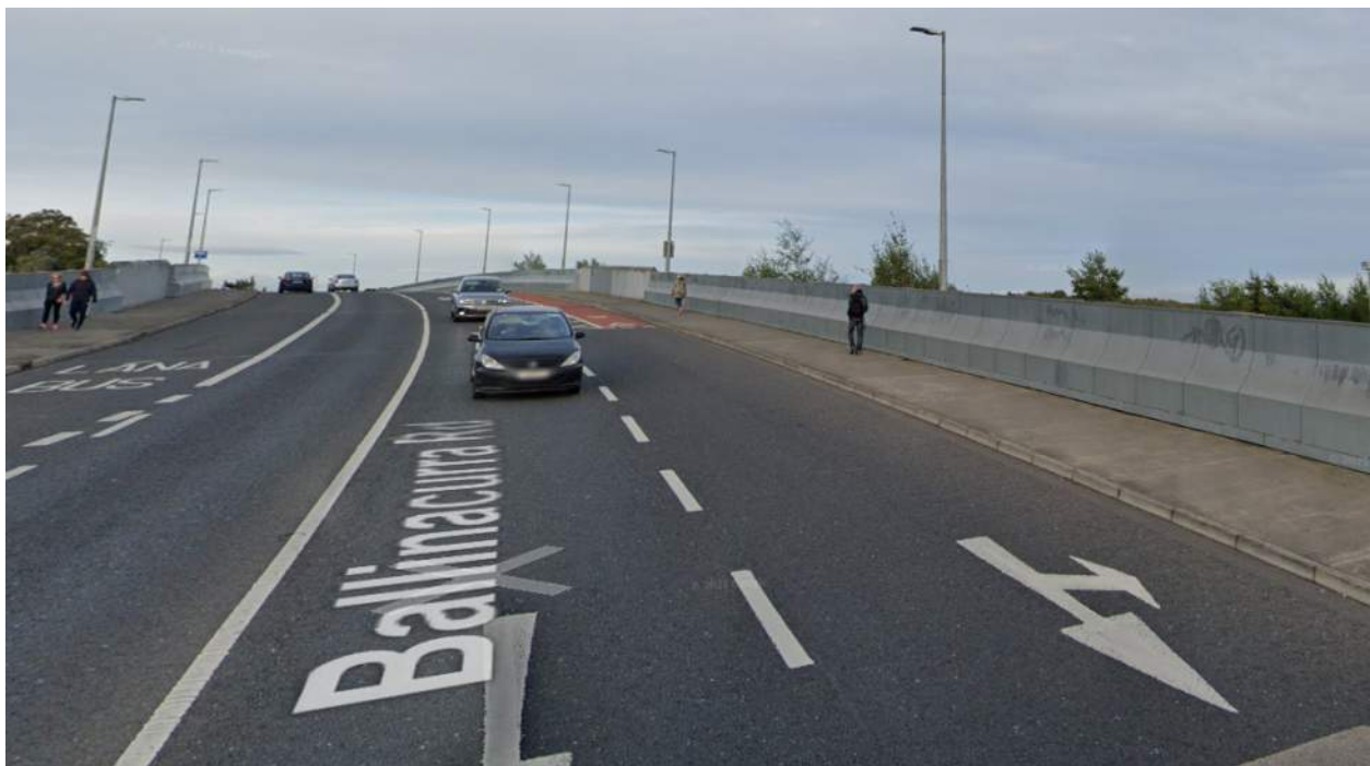
Figure 5-4: Image of Existing At-Grade Cycle Track ending at left turn lane for Crescent Shopping Centre (© Google)
