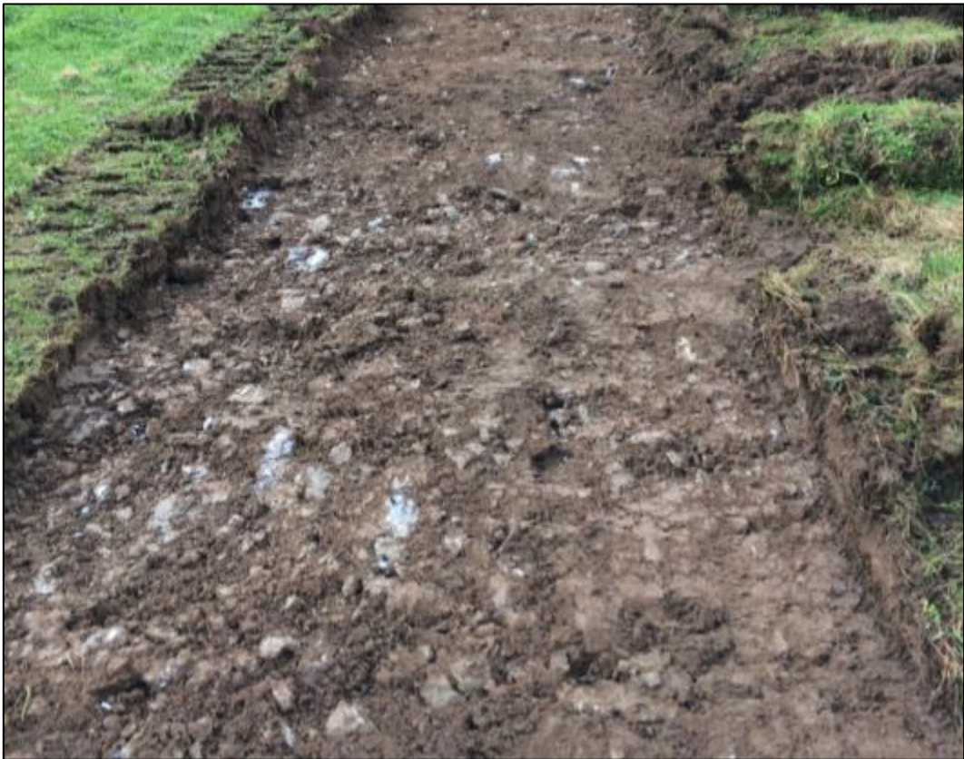
Plate 4: View of stone track in Trench 2
