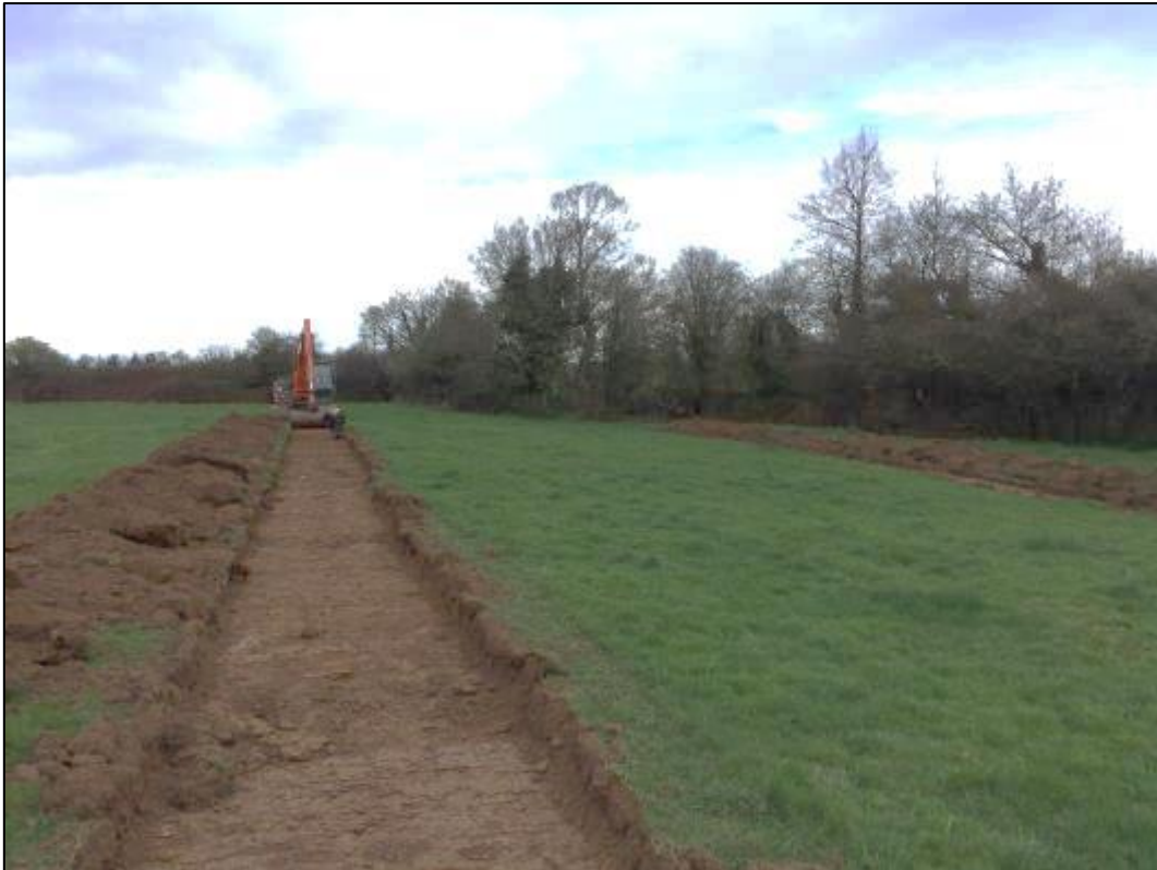
Plate 7: View of excavation of Trench 4 from south
