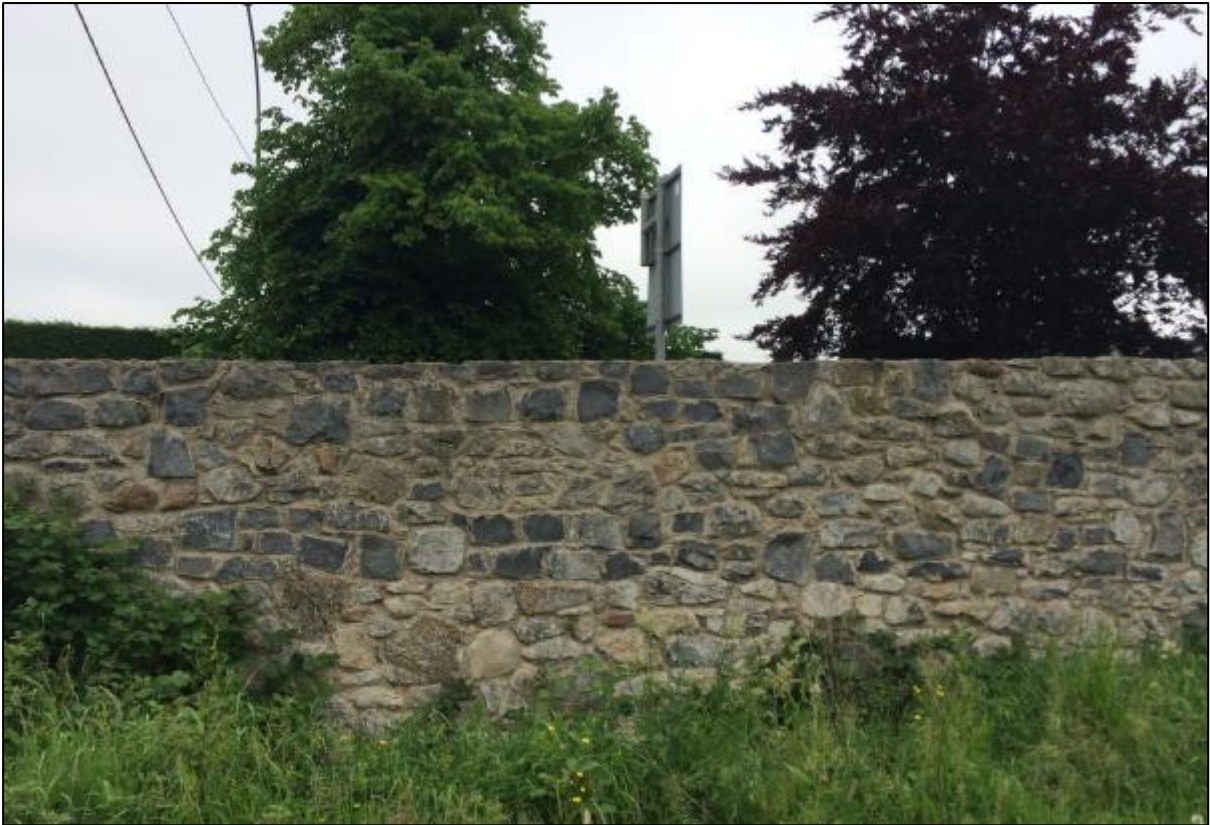
Plate 9: View of rebuilt southern boundary wall
