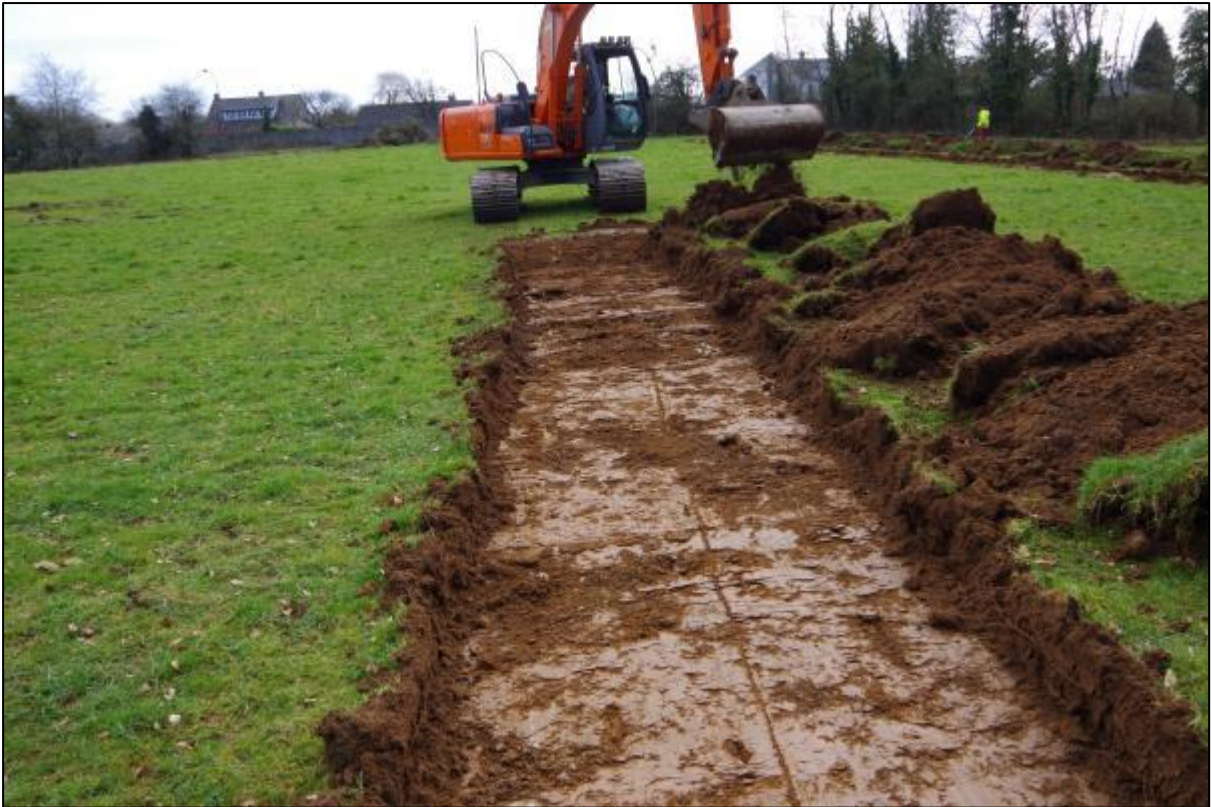
Plate 5: View of excavation of Trench 4 from north
