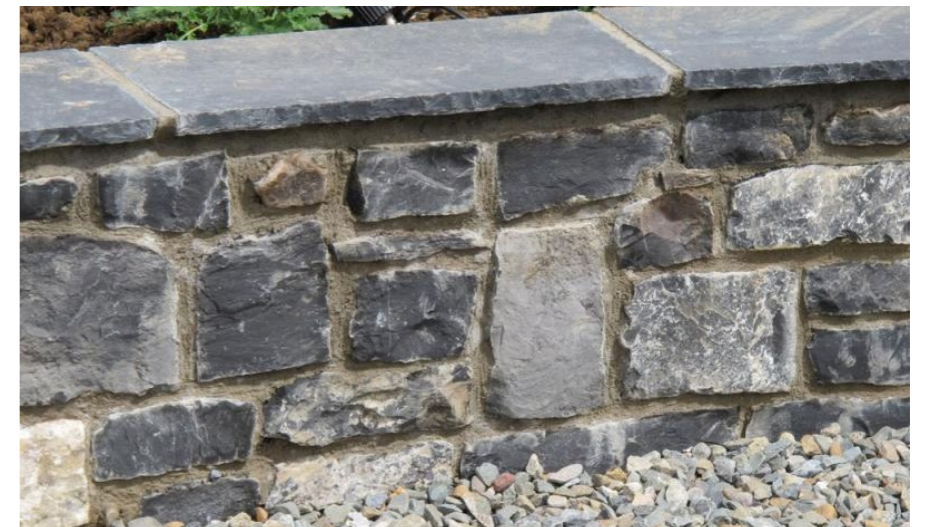
Raised beds within public open space and car park to use limestone walls to match existing boundary walls
