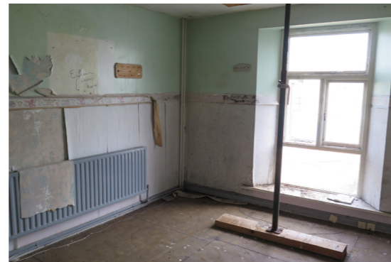
Photo 10: Second Floor Rear Room
