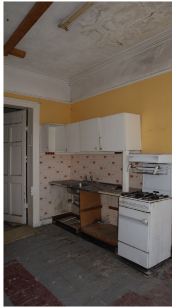
Photo 17: First Floor Front Room
