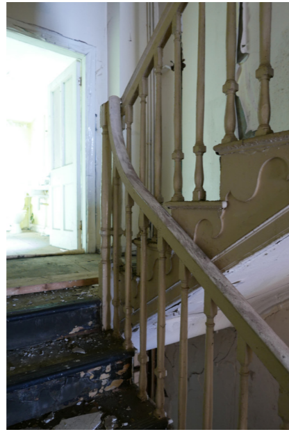
Photo 18: Second Floor Half Landing
