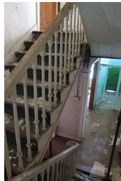
Photo 30: First Floor Half Landing
