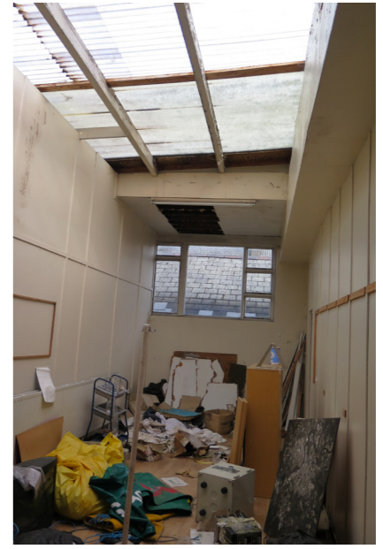
Photo 22: Former Firestation Building First Floor Rear Store
