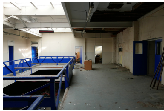
Photo 24: Former Firestation Building First Floor
