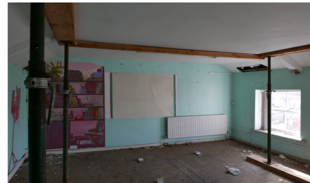
Photo 11: Third Floor Front Room
