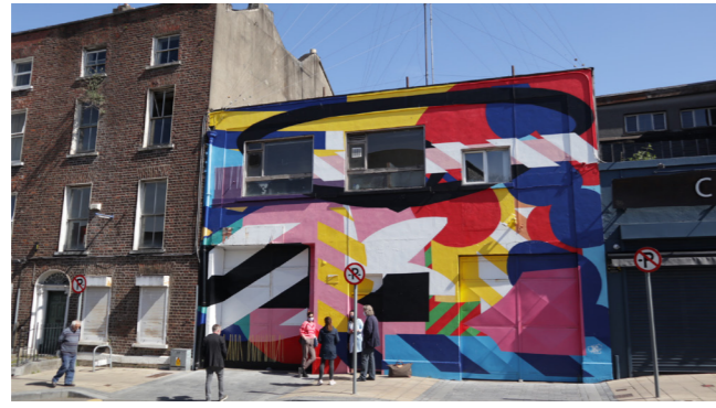
Photo 01: Front Elevation of No. 33 & 34 Thomas Street
