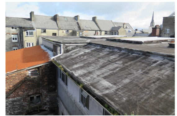
Photo 26: View of No. 34 Thomas Street
