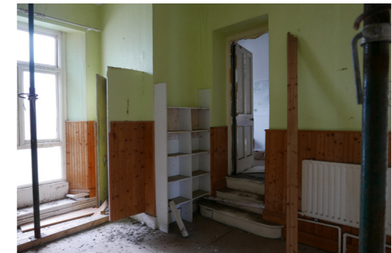
Photo 08: First Floor Rear Room
