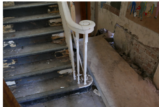
Photo 05: Staircase Original Handrail and Baluster
