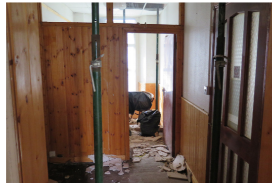
Photo 06: Ground Floor Modern Partitions in Rear Room
