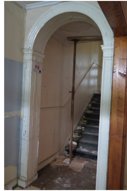
Photo 20: Ground Floor Entrance Hall
