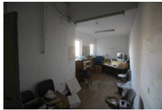
Photo 25: Former Firestation Building First Floor Office
