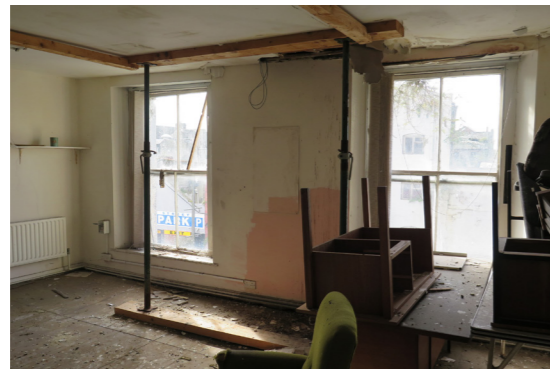
Photo 09: Second Floor Front Room
