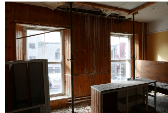
Photo 07: First Floor Front Room
