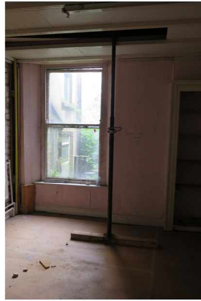
Photo 19: Ground Floor Rear Room
