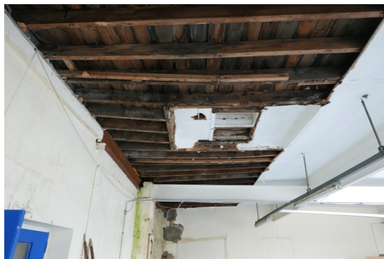
Photo 23: Former Firestation Building First Floor Roof Joists
