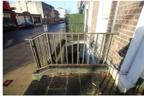
Photo 02: Lightwell to front of No.32 Thomas Street
