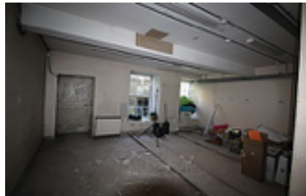
Photo 25: Basement Front Room
