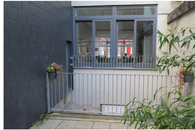
Photo 33: Aluminum Window to be Retained at Ground Floor
