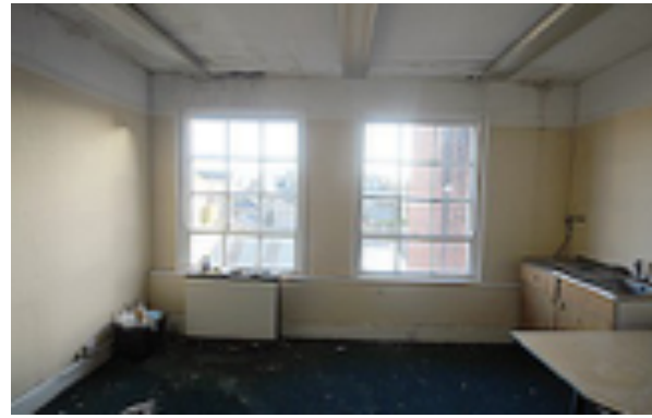
Photo 17: Original Sash Windows in Third Floor Rear Room
