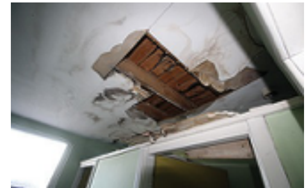
Photo 24: Opening-up Works in Rear Return
