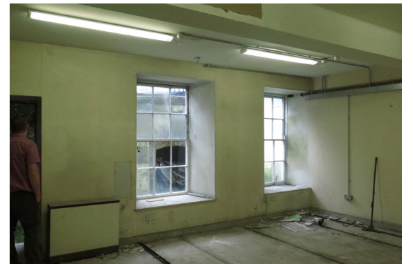
Photo 26: Original Sash Windows in Basement Front Room
