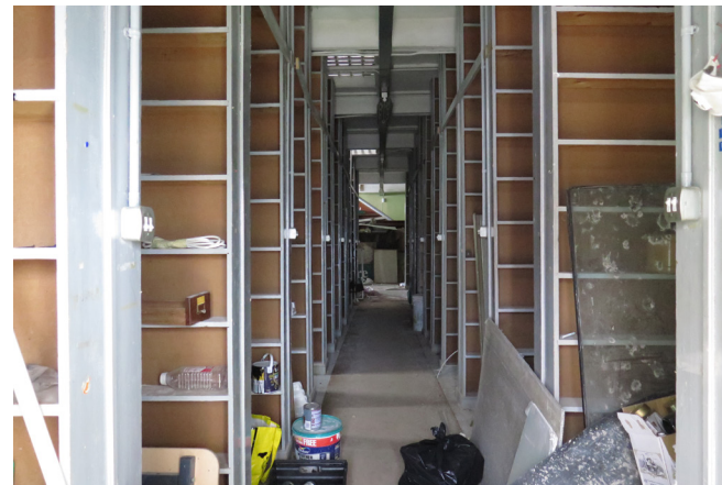
Photo 36: Shelving in Library Store / Warehouse Building
