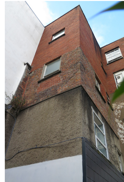
Photo 42: View of Rear Return
