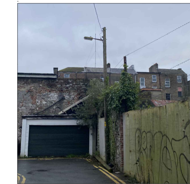
IMAGE C (POLE TO BE RETAINED, LIGHT FITTING TO BE REPLACED WITH NEW LED TYPE LUMINIARE)
