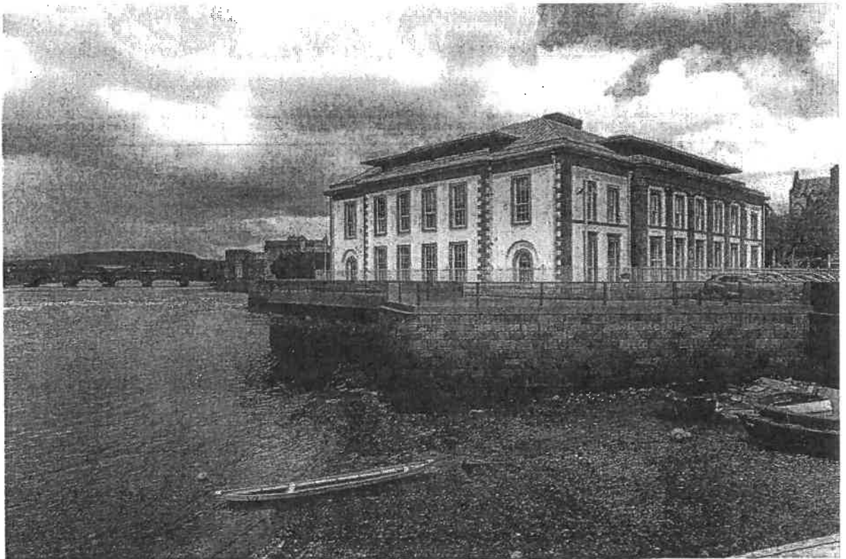
Fig. From developer's photomontage post flood relief works showing quay wall near Court devoid of bryophytes vegetation which required centuries to establish
