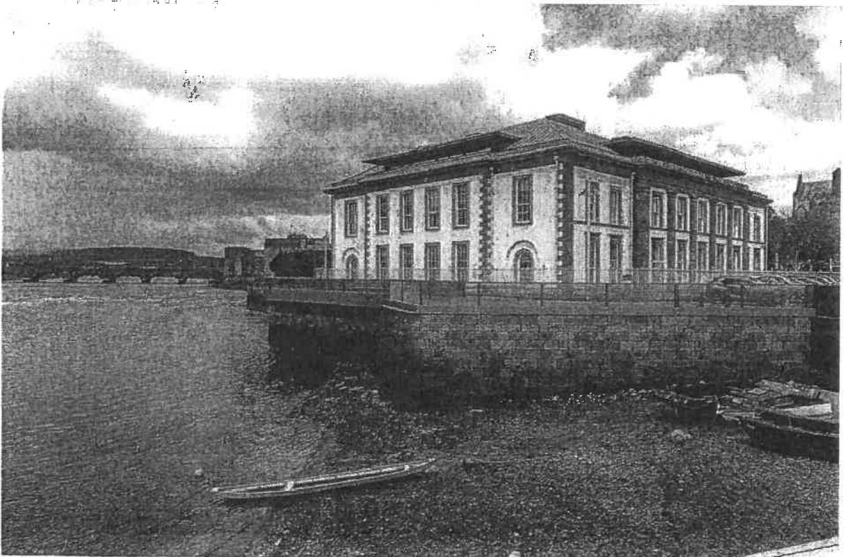
Fig. From developer's photomontage post flood relief works showing quay wall near Court devoid of bryophytes vegetation which required centuries to establish
