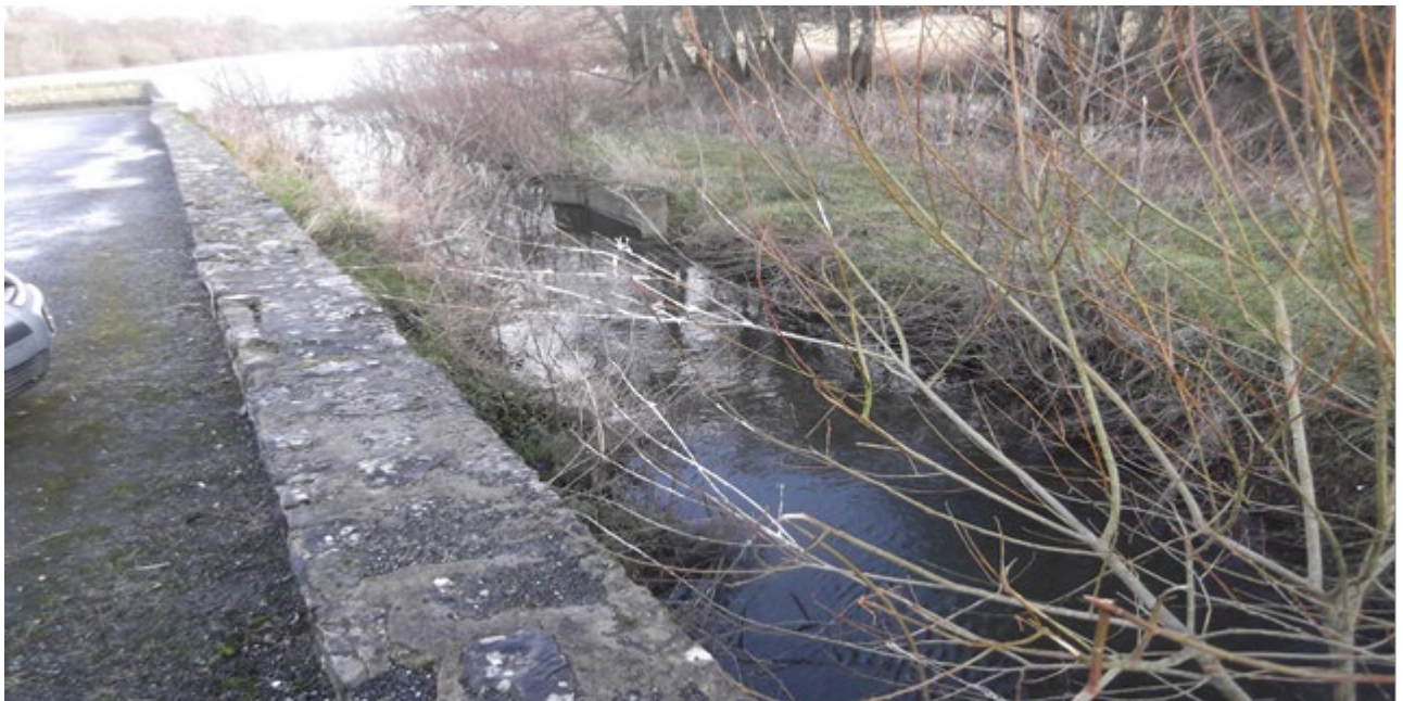
Figure 2: Channel entering the river at Ferrybank
