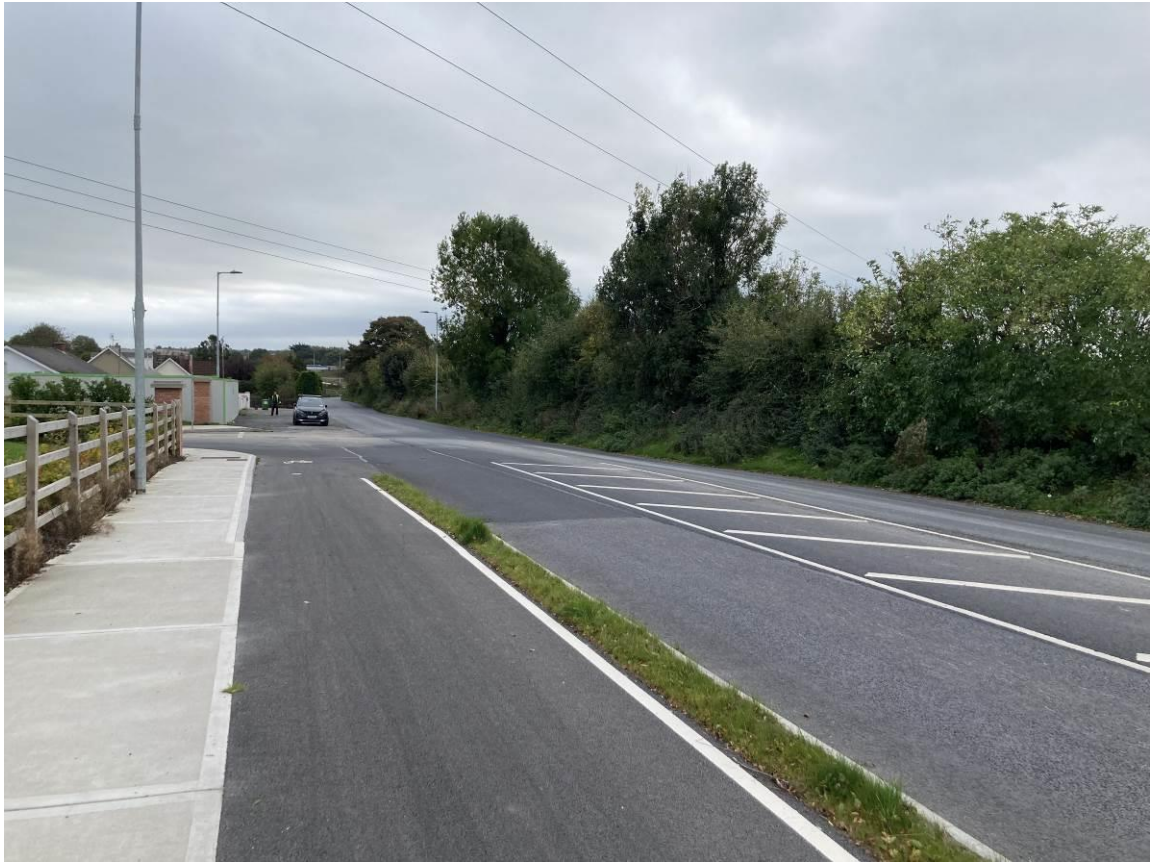
Photo A2: Tie in location at Western extent of scheme
