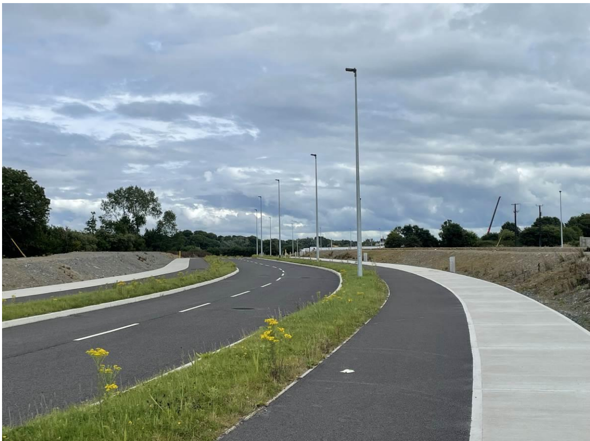
Photo A1: Existing Link Rd at Eastern Extent of scheme
