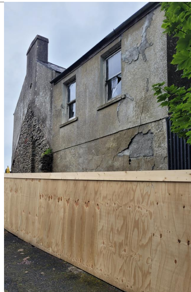
Image 4-2: View of the building from the north.
