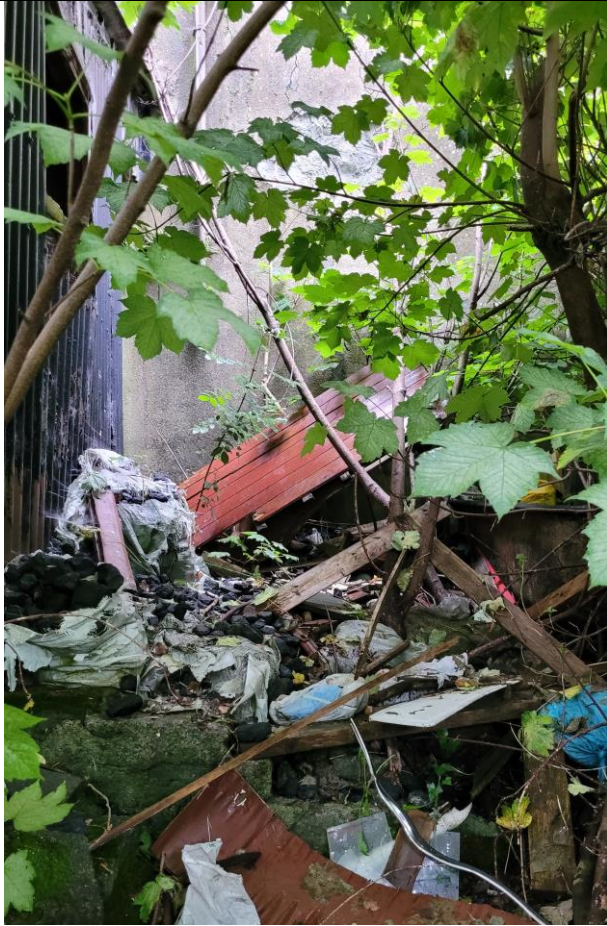
Image 4-3: Waste material dumped at the rear of the house.
