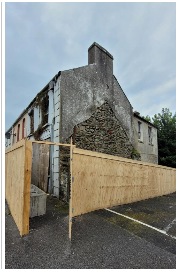
Image 4-1: View of the building from the front (east).
