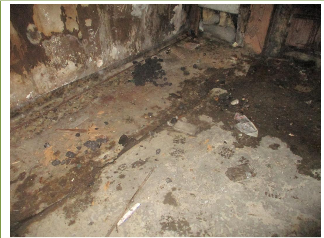
Floor covering in the ground floor kitchen
