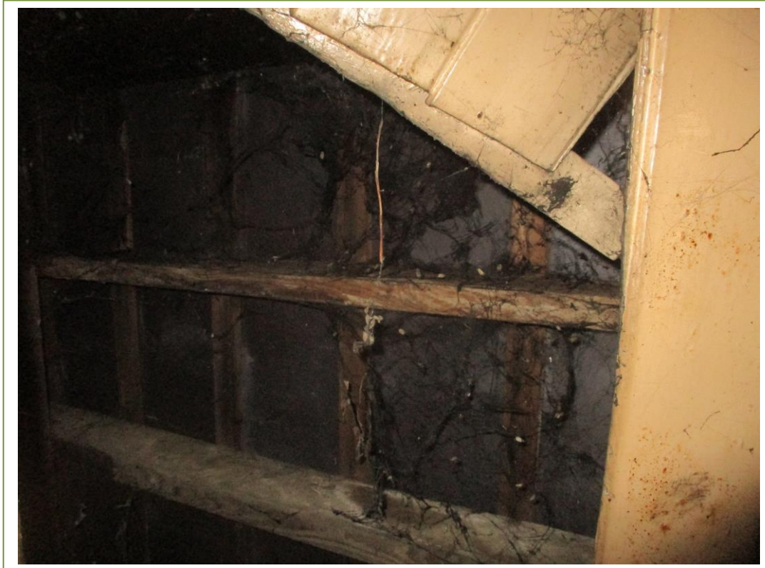
Natural slates on the main roof
