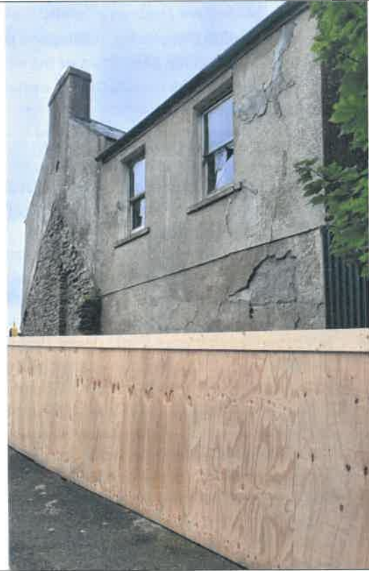
Image 3-2: View of the building from the north.
