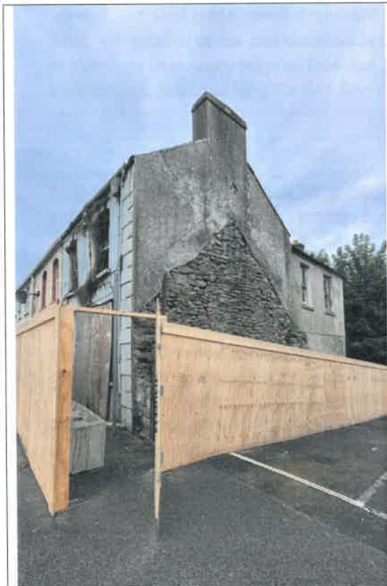
Image 3-1: View of the building from the front (east).
