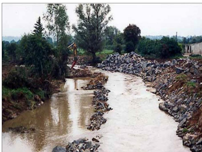
Plate 6 River drainage and modification works have impacted the Kileengarrif River in the past. OPW arterial drainage works on the Kileenagarrrif River during 1996.
