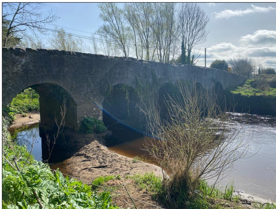
Plate 1 Kileengarriff Bridge during March 2021.
