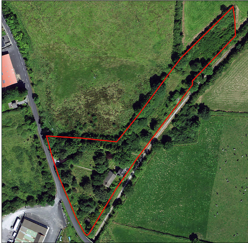
Figure 5. Aerial view of Ardagh Train Station, prior to renovation (after Digital Globe 2011). North to top.
