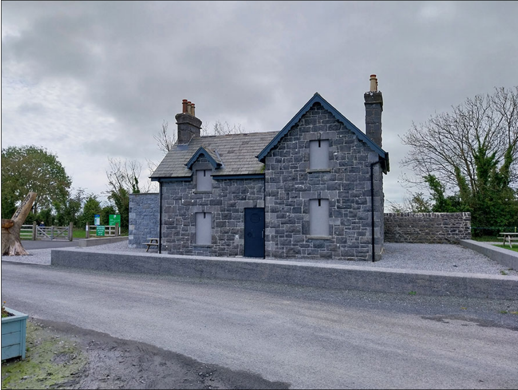
Plate 1. View of rear of Station House, from car park at W.
